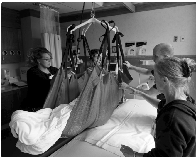
At PeaceHealth in Eugene, Oregon, ceiling mounted lifts were installed on two units to test their effectiveness and safety with patient-handling activities. The pilot was so successful, reducing staff back injuries by 83 percent, that the design feature was adopted hospital-wide, according to a March 2006 article in Healthcare Design Magazine .
