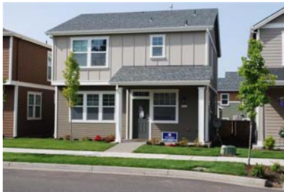
Privately owned house at New Columbia
