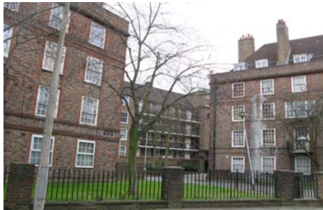
Existing council housing at Clapham Park
