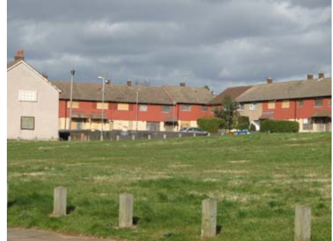
Existing council housing at Wood End
