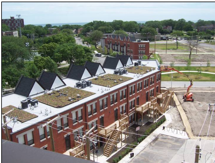
Construction at Oakwood Shores, including green roofs
