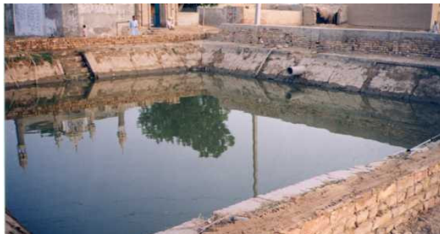
Community storage tank for domestic use of irrigation water, Pakistan.
