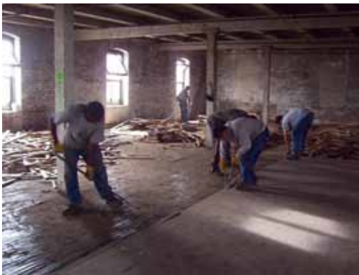
Workers for The ReUse Center engage in salvage operation while deconstructing a building. Photo courtesy of The ReUse Center
