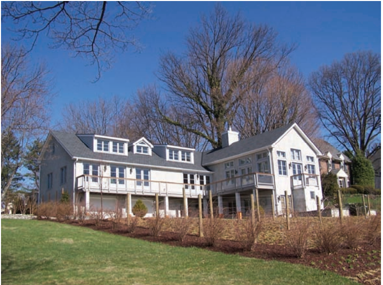
This home in the Borough of Doylestown, PA was constructed using the Borough's Green Points program. The project saved more than one thousand dollars in permit fees. SOURCE: Doylestown Borough Planning Commission
