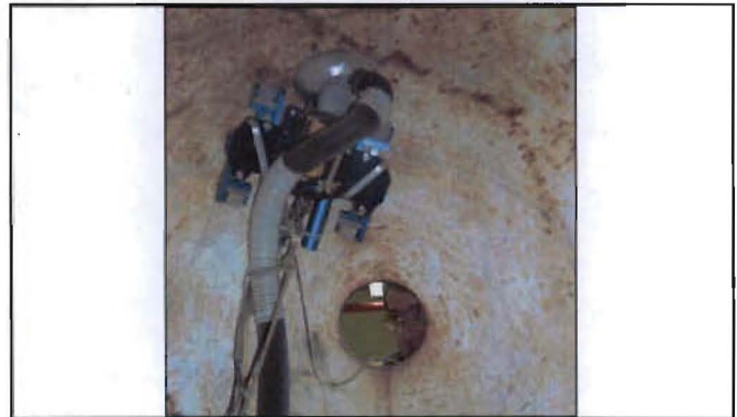
Figure 12. Crawler brushing inside a vessel.
