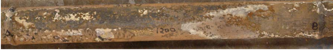
12 O'Clock – Facing Gas Flow (Note: 3 o'clock is up in this image)
