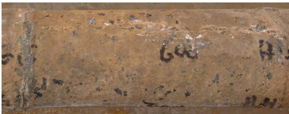
6 O'Clock – Opposite Gas Flow
