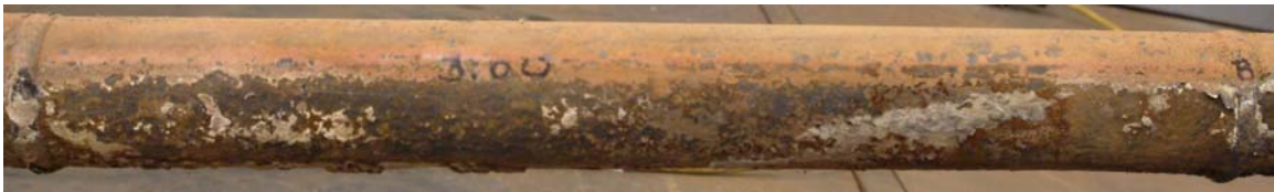
3 O'Clock (Note: 6 o'clock is up in this image)
