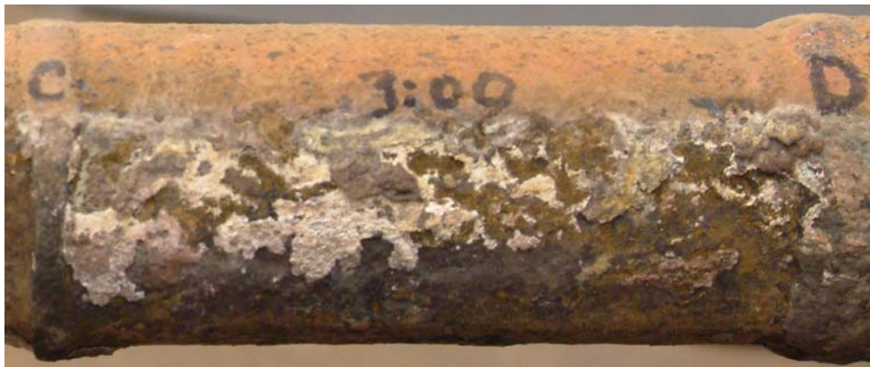
3 O'Clock (Note: 6 o'clock is up in this image)
