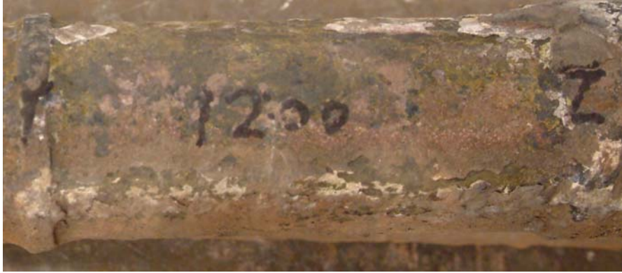
12 O'Clock – Facing Gas Flow (Note: 3 o'clock is up in this image)
