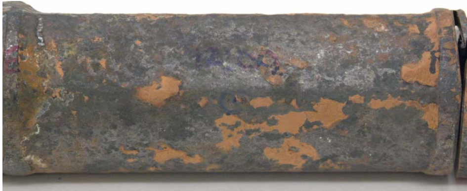
12 O'Clock – Facing Gas Flow (Note: 3 o'clock is up in this image)
