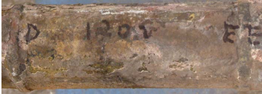
12 O'Clock – Facing Gas Flow (Note: 3 o'clock is up in this image)
