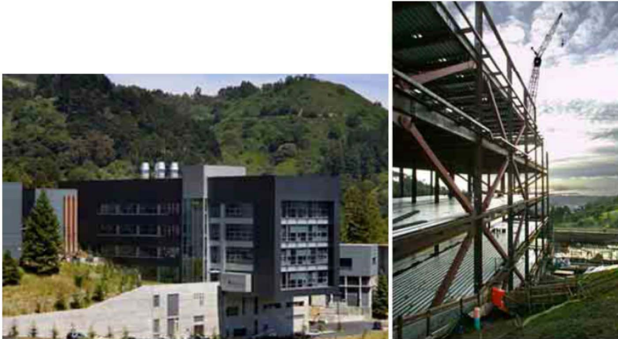
Figure 4. Experimental test site. Left: the Molecular Foundry building at LBNL. Right: view of the building during construction revealing the steel decks between floors.
