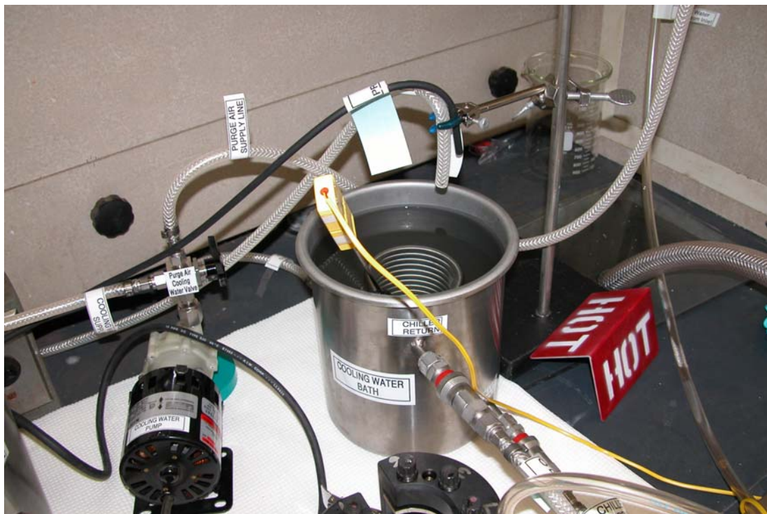
Figure 2-5. Portion of the first cooling water system.
