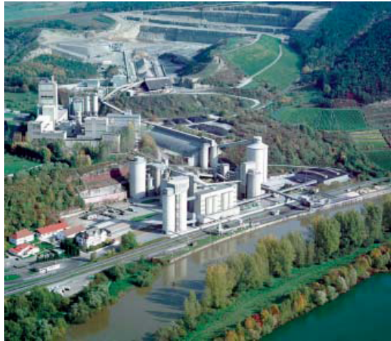
1.5 MW Ormat ® Energy Converter at the Lengfurt Cement, Germany, image taken from http://www.ormat.com/FileServer/70b593358e2da845c512c50dc0c47613.pdf
