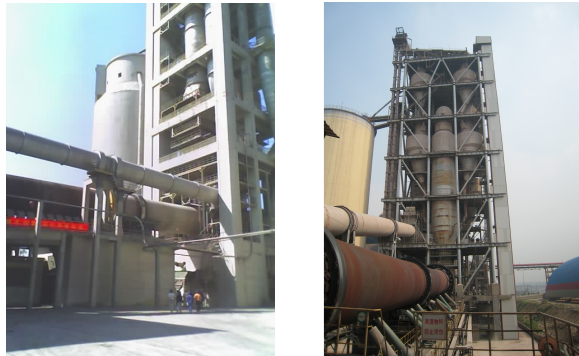
Sample images from Chinese cement plants having rotary kilns with preheaters and precalciners.
