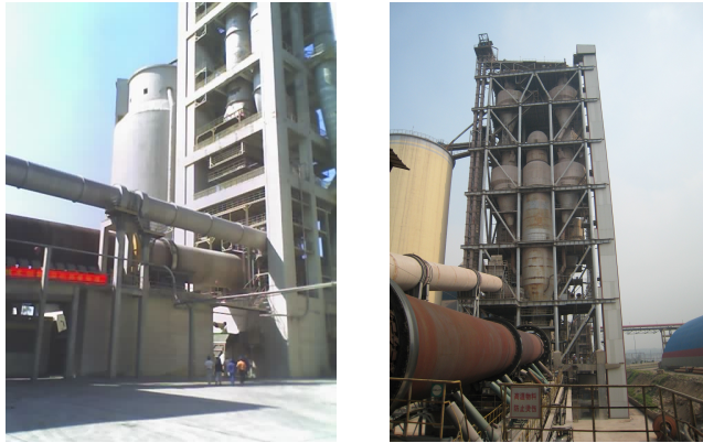
Sample images from Chinese cement plants having rotary kilns with preheaters and precalciners.
