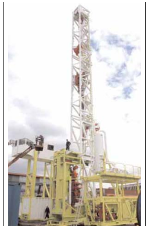
Figure 30. Huisman Rig during rig-up.
