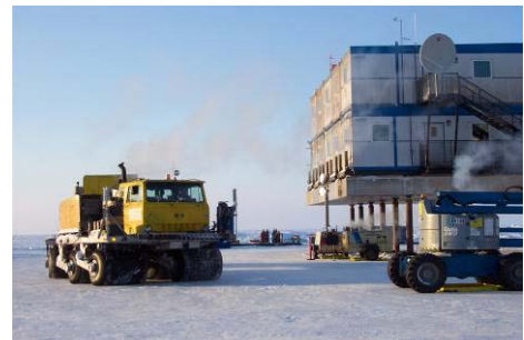
Figure 21. Rolligon during platform installation.
