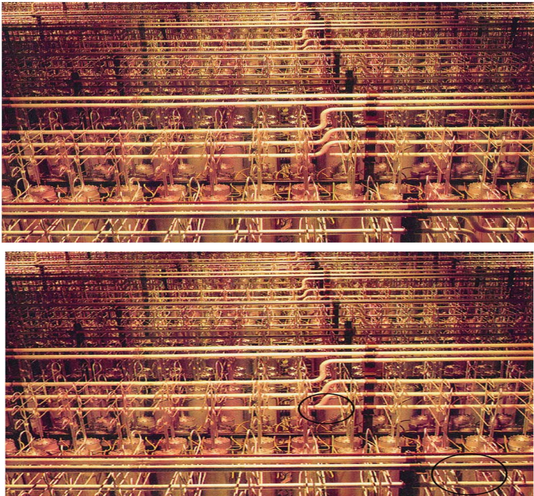
Figure 9: Comparison of Reference Photo for Enrichment Cascade Hall with Altered Image Using Change Detection Software
