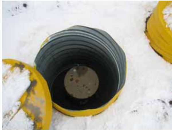
Figure 2.2. Typical Instrument Surface Completion Showing Outer 24-In.-Diameter Corrugated Metal Pipe Sleeving and Inner Steel Casing (Nest A; photo taken in the winter 2008; snow can be seen on the ground)
