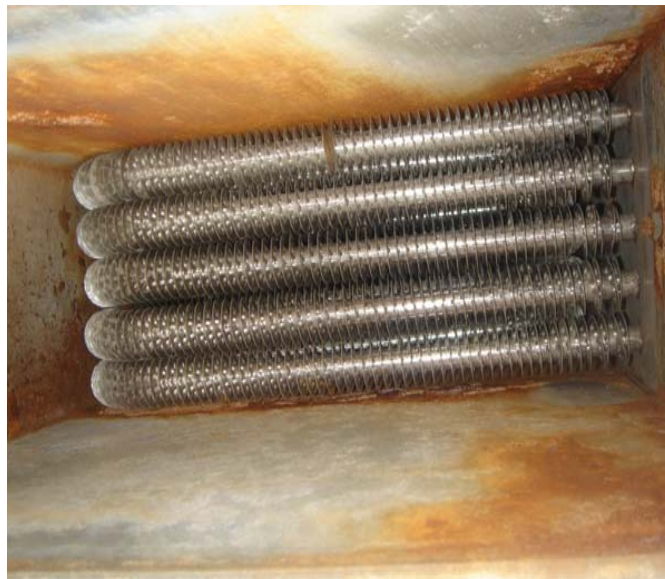
Figure 2-4: Fin-Tube Heat Exchanger Bundle Mounted in Duct.
