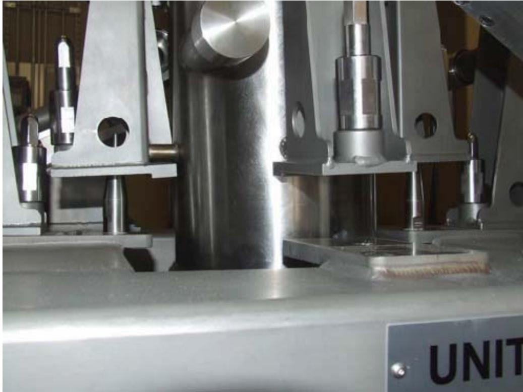
Figure 14 Close up view of guide pins during contactor unit installation
