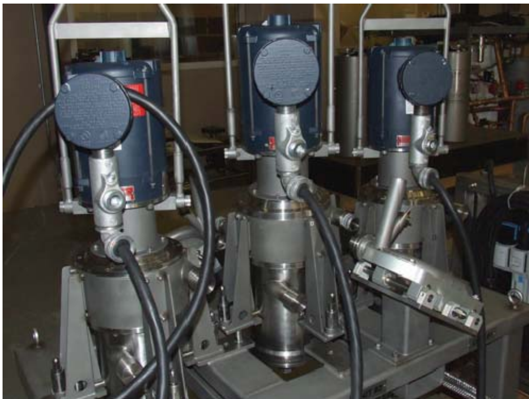
Figure 13 Re-installation with guide pins halfway engaged
