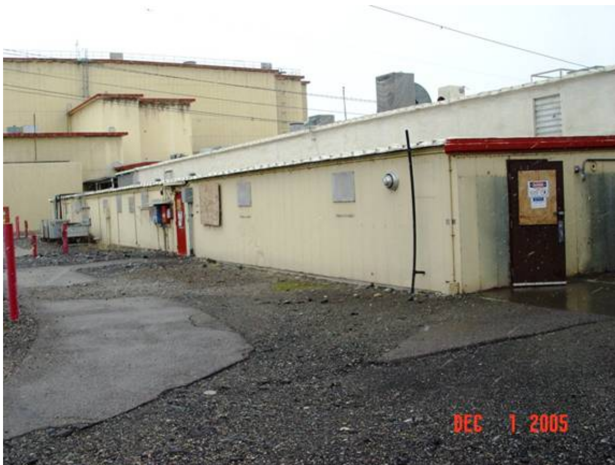
Figure 18. 1705-NA Maintenance Shop Annex.
