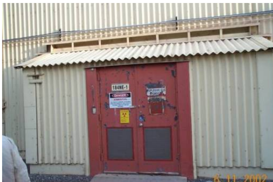
Figure 12. 184-NE-1 Compressed Gas Shed.
