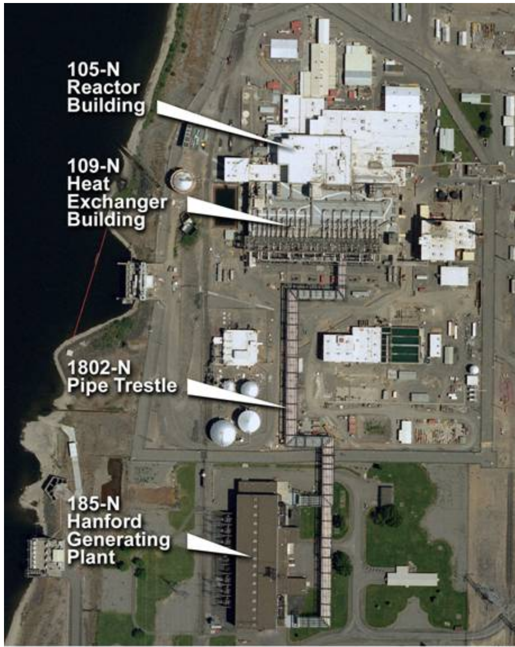
Figure 24. 1802-N Pipe Trestle.
