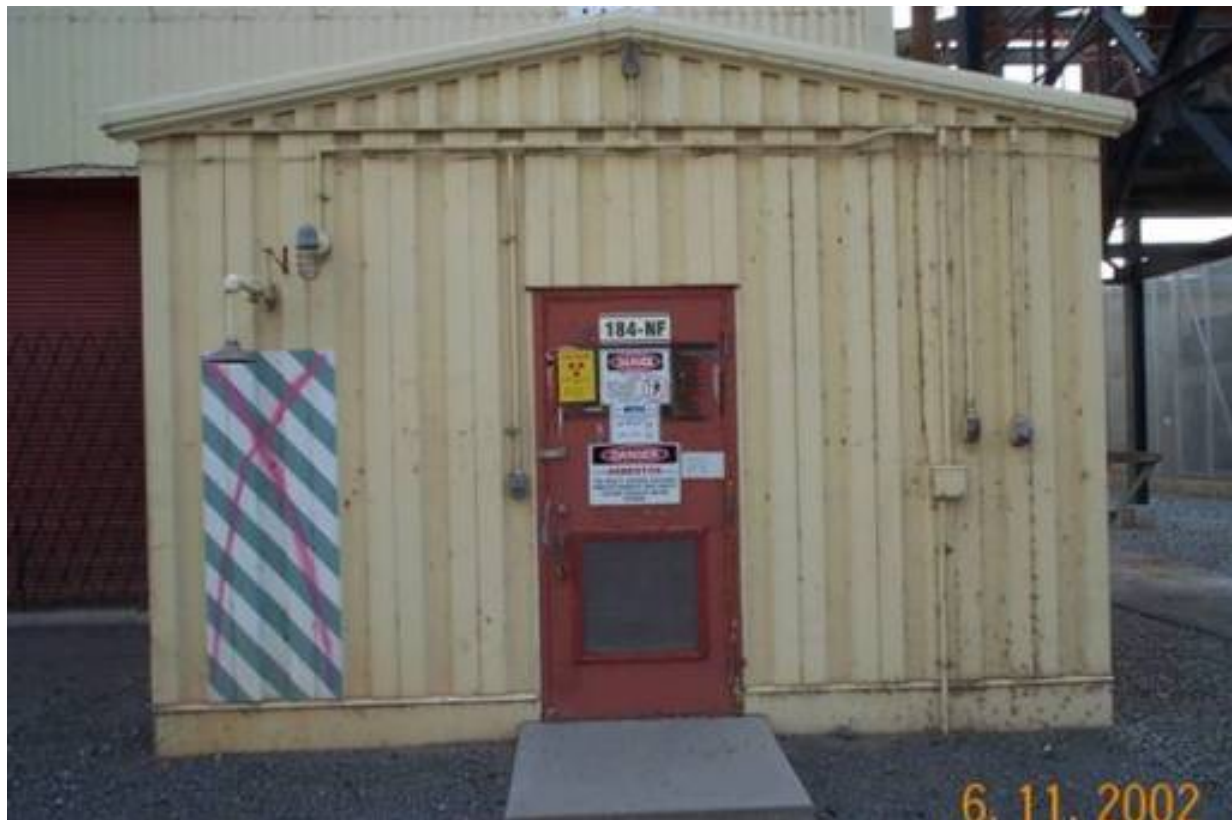
Figure 14. 184-NF Chemical Injection Pump Shed.
