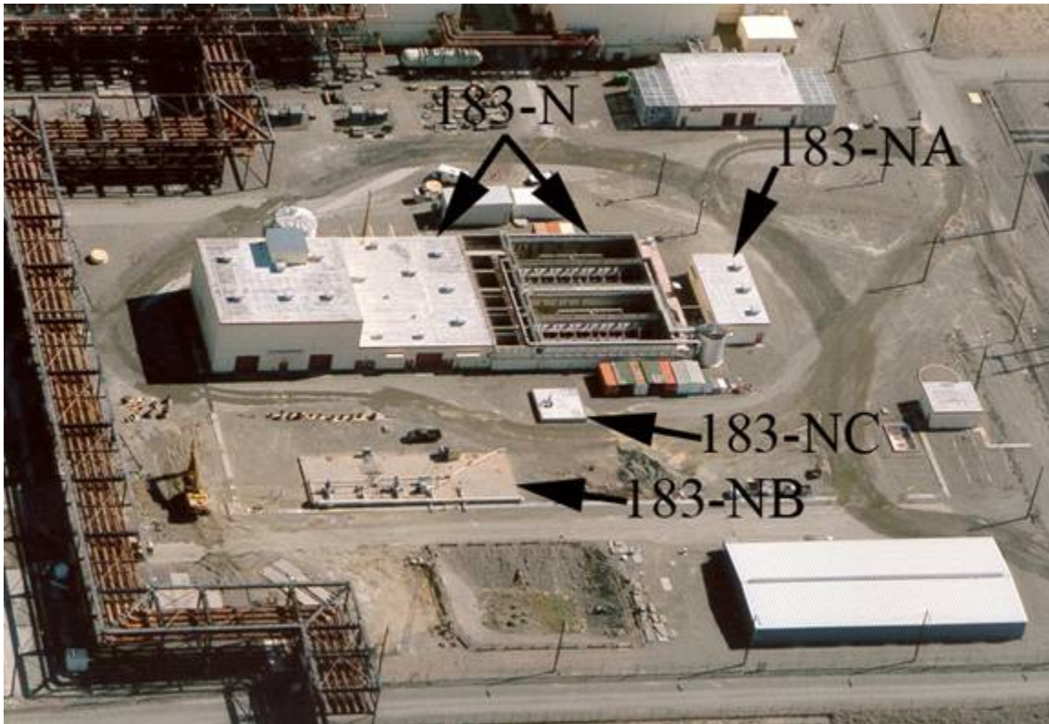
Figure 3. 183-N Water Filter Plant.
