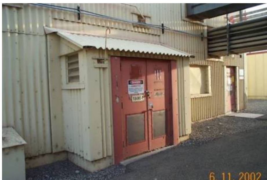
Figure 13. 184-NE-2 Compressed Gas Shed.
