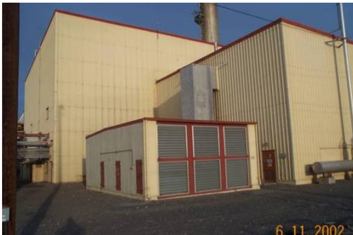
Figure 10. 184-NC Air Handling Annex Building.
