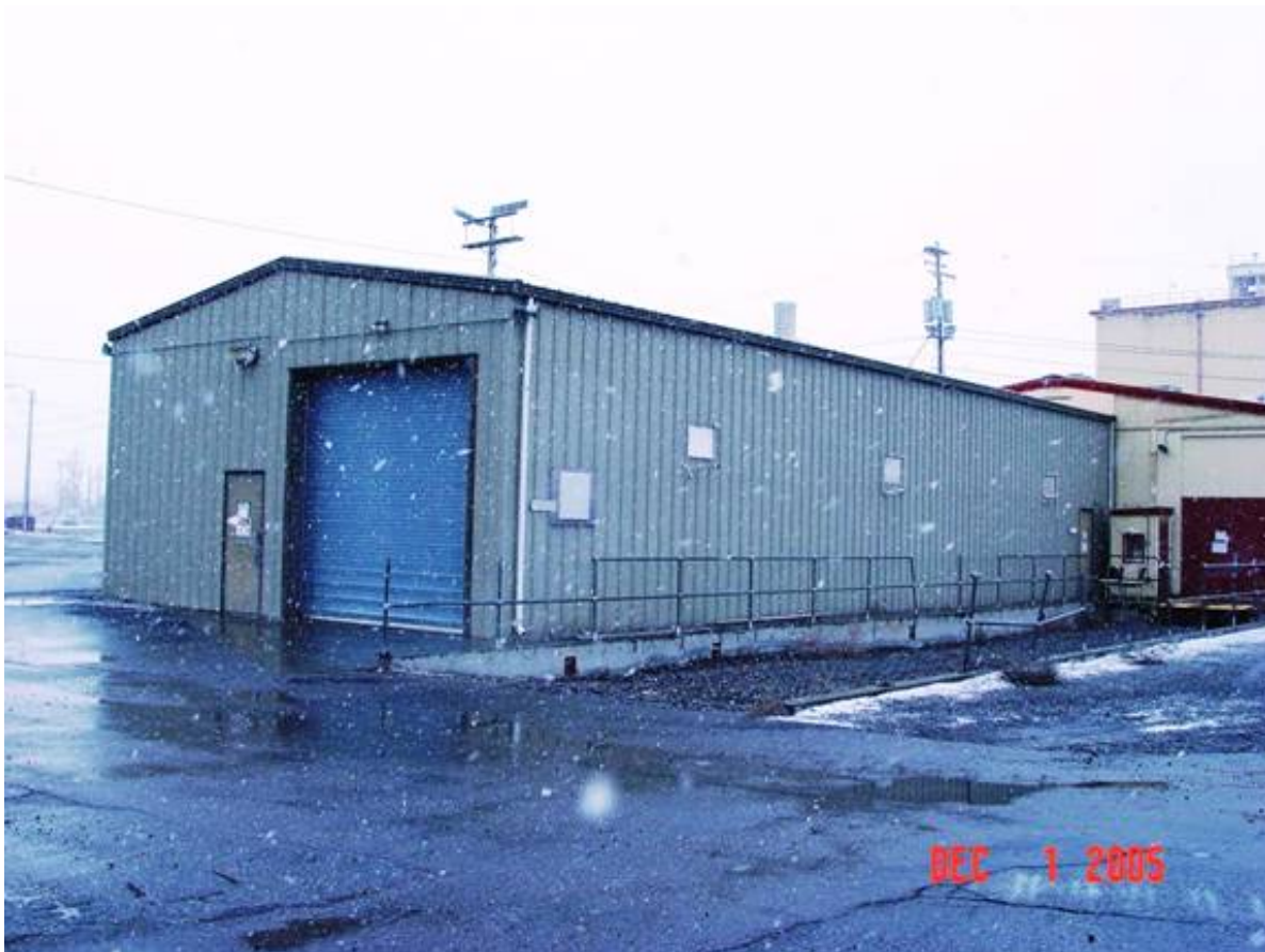
Figure 19. 1706-N Storage Building/Maintenance Shop.
