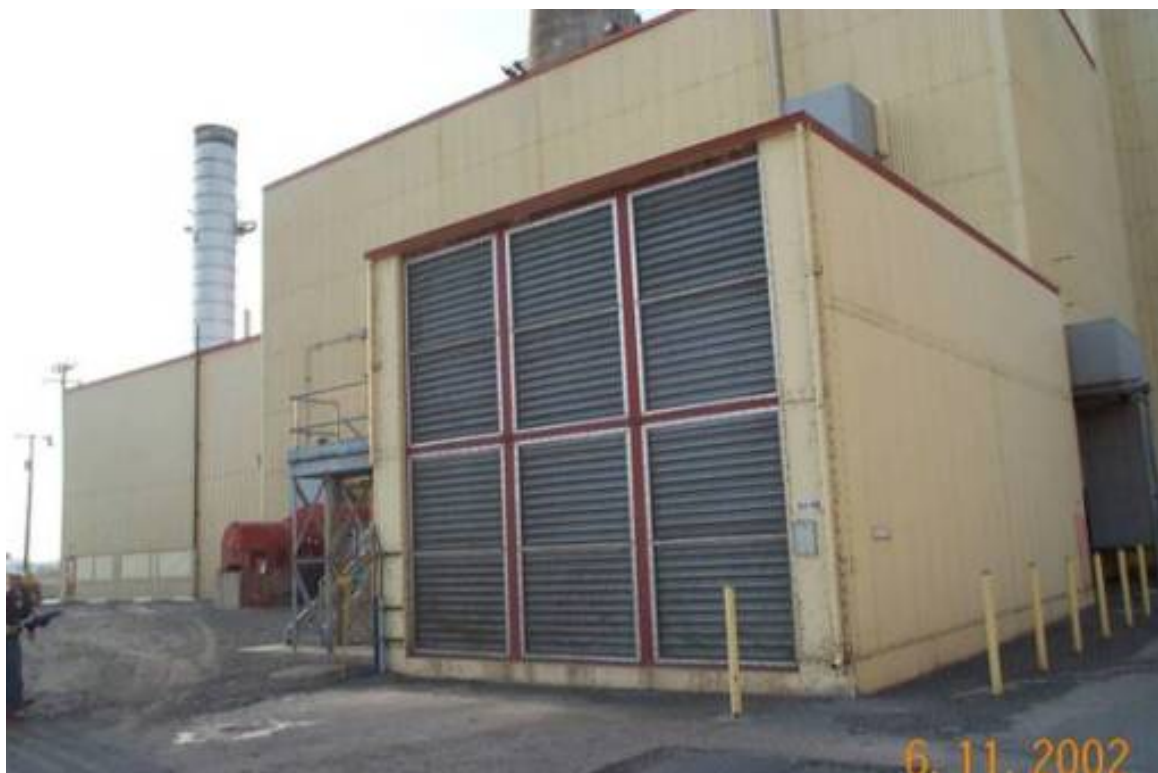
Figure 9. 184-NB Air Handling Main Building.
