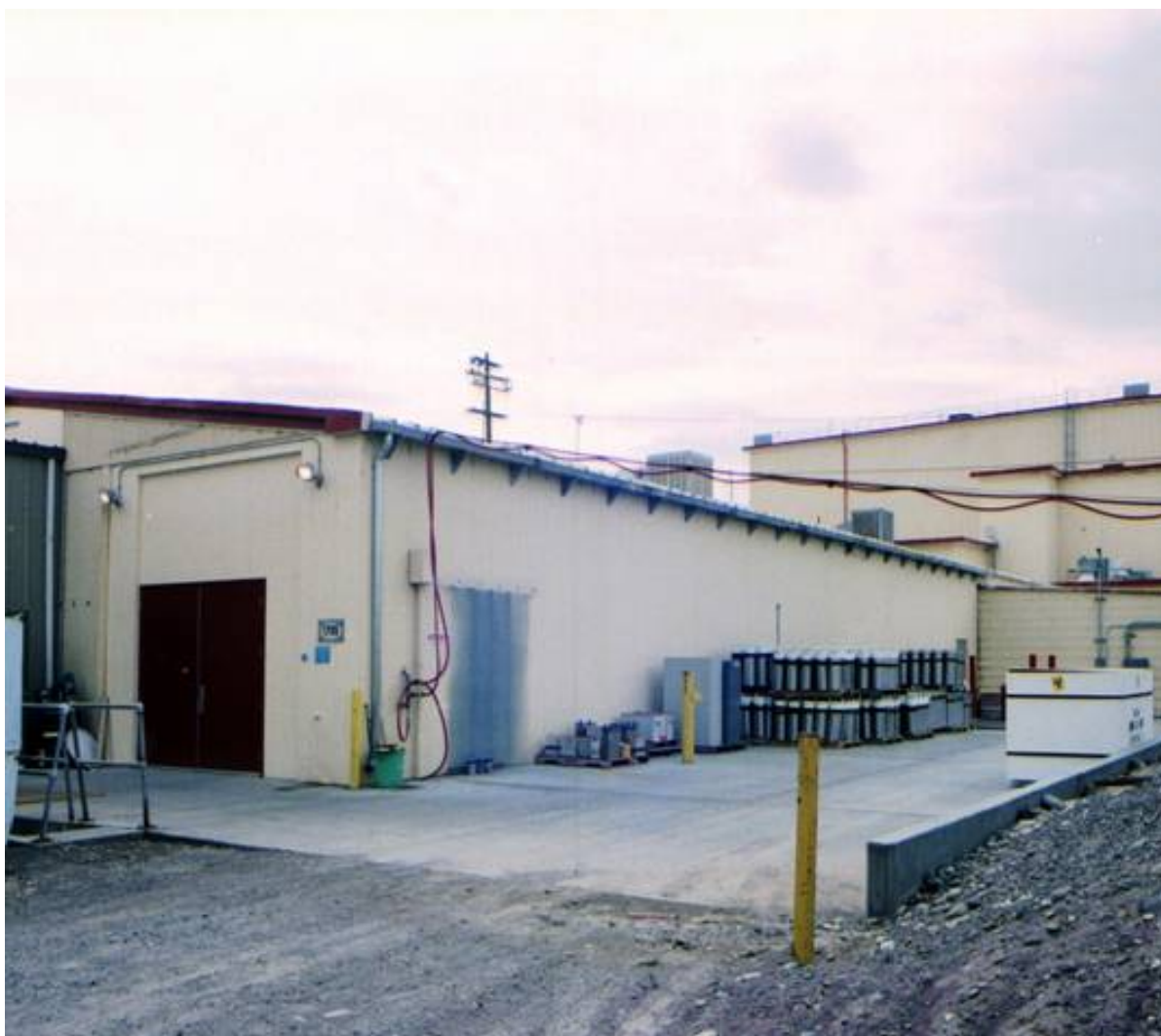
Figure 17. 1705-N Instrument and Electrical Facility.
