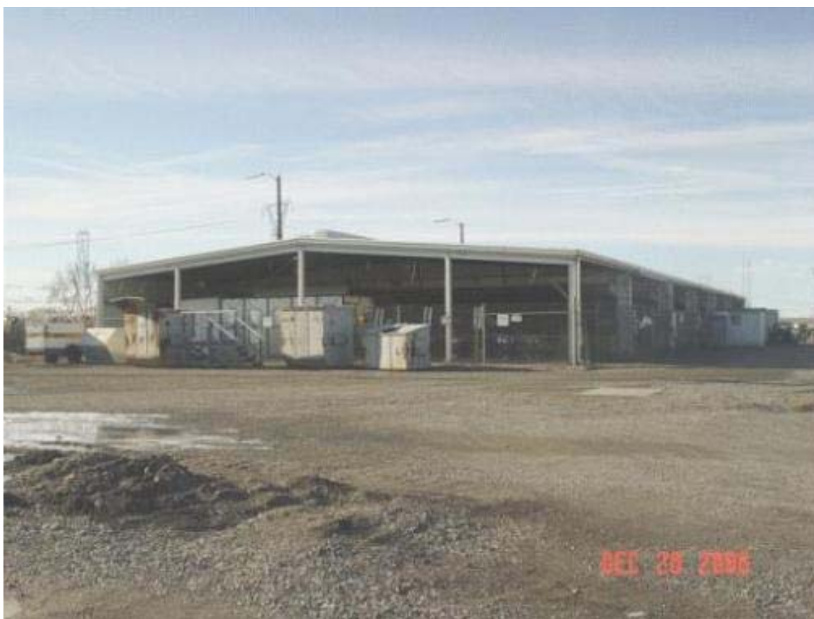
Figure 16. 1330-N Waste Storage Facility.
