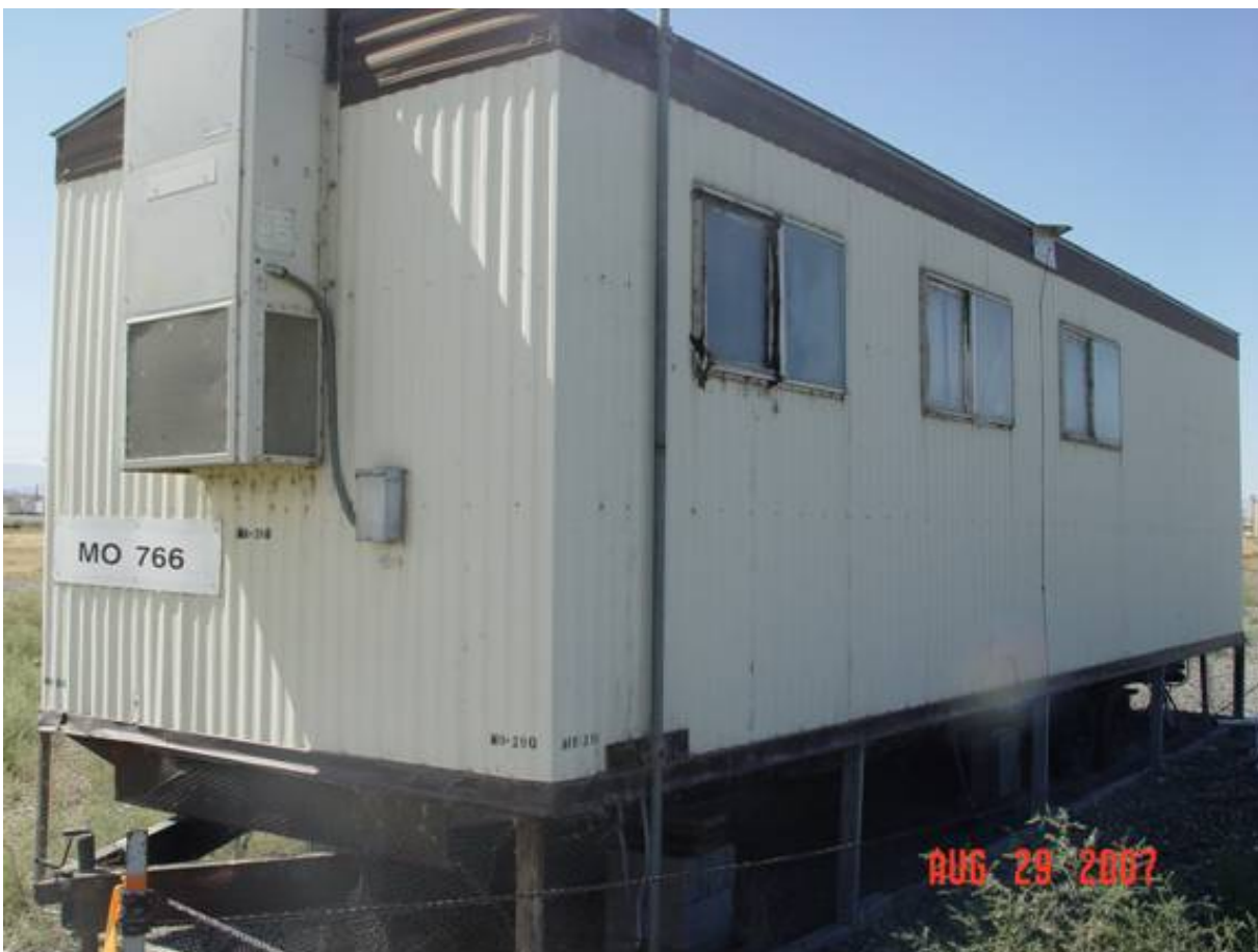
Figure 28. MO-390 Mobile Office (Field Trailer).
