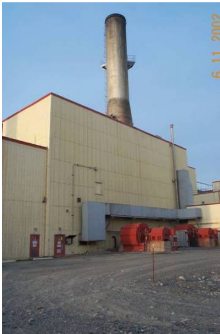
Figure 7. 184-N Plant Service Power House.
