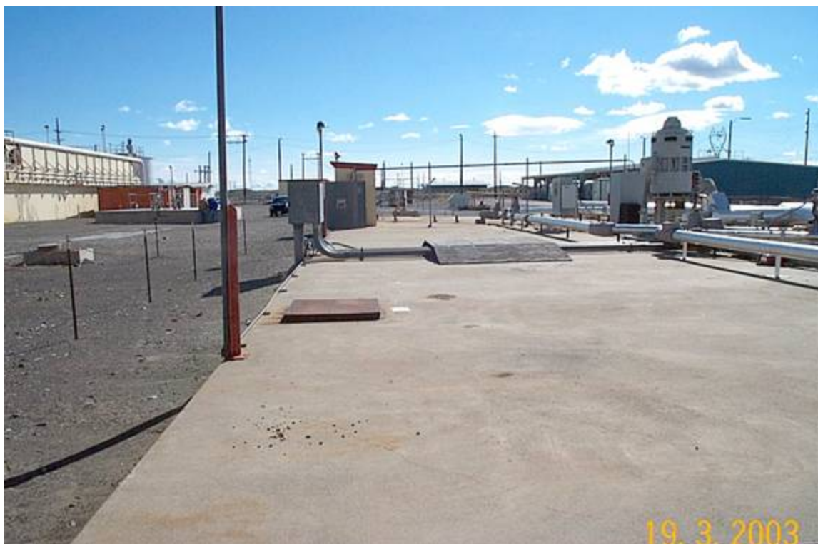
Figure 5. 183-NB Water Filter Plant Pump House.
