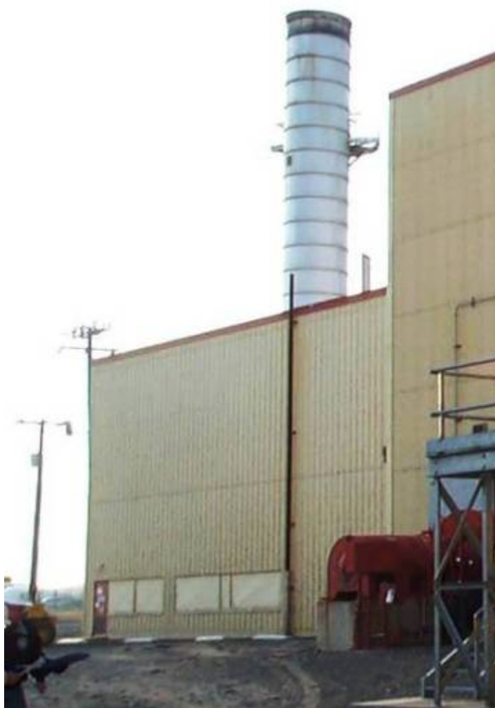
Figure 8. 184-NA Auxiliary Power Annex Building.
