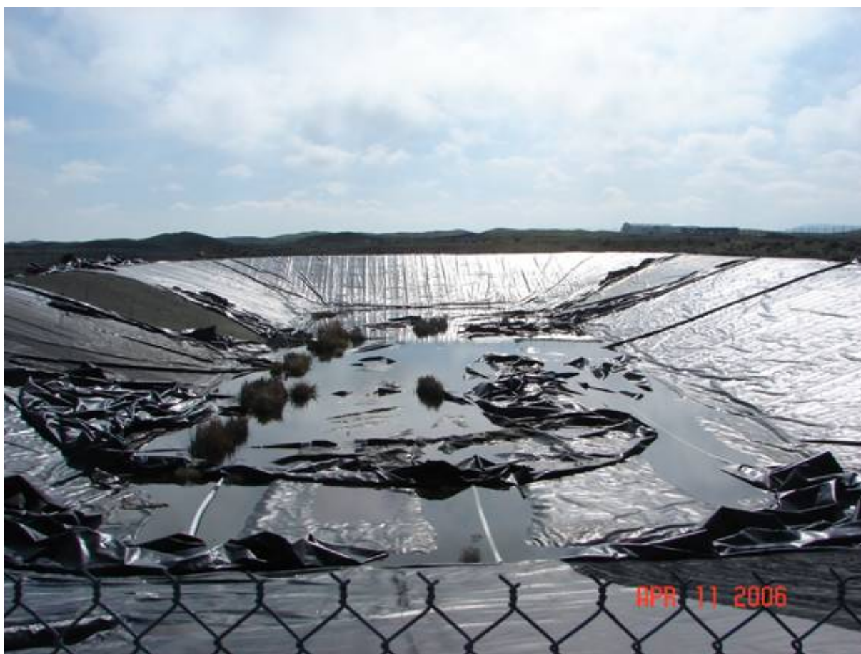
Figure 15. 1312-N Liquid Effluent Retention Basin.
