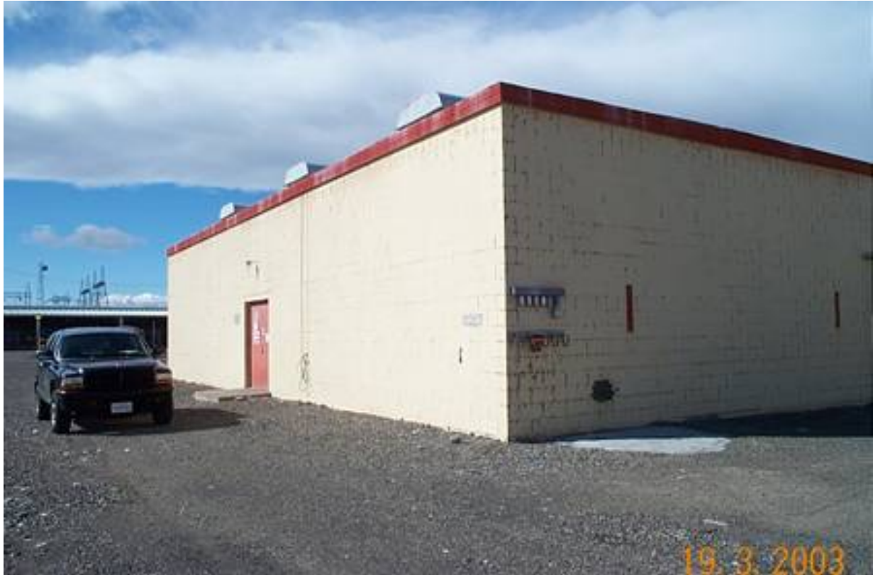
Figure 4. 183-NA Water Filter Plant Pump House.
