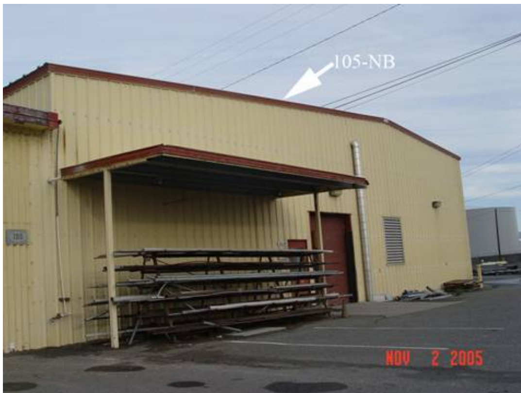
Figure 1. 105-NB Maintenance Building Addition.
