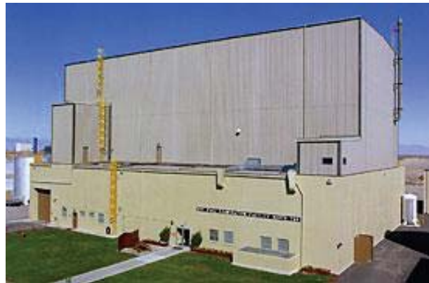
Figure 1. Hot Fuel Examination Facility at MFC.
