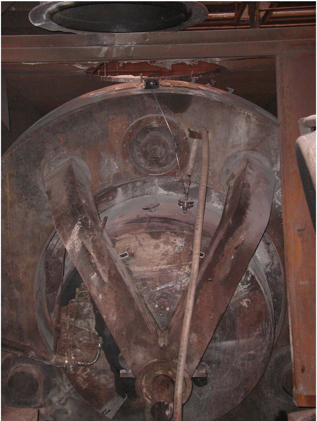
Figure 8 Initial tuyere installation in the Universal Converter
