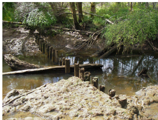
Figure G.8. Cross Sections at Deep River. (a) Cross sections 25.4 m upstream of the centerpoint of the former dike showing flushing of organic matter after dike breaching in 2005; (b) pilings that formed the inner wall of the dike at the mouth of the channel on Deep River were removed to the level of mineral soil at the time of dike breaching in 2005; (c) 1.5 years later, the channel mouth has incised 2.86 m as measured by the same pilings, which were excavated by channel processes.
