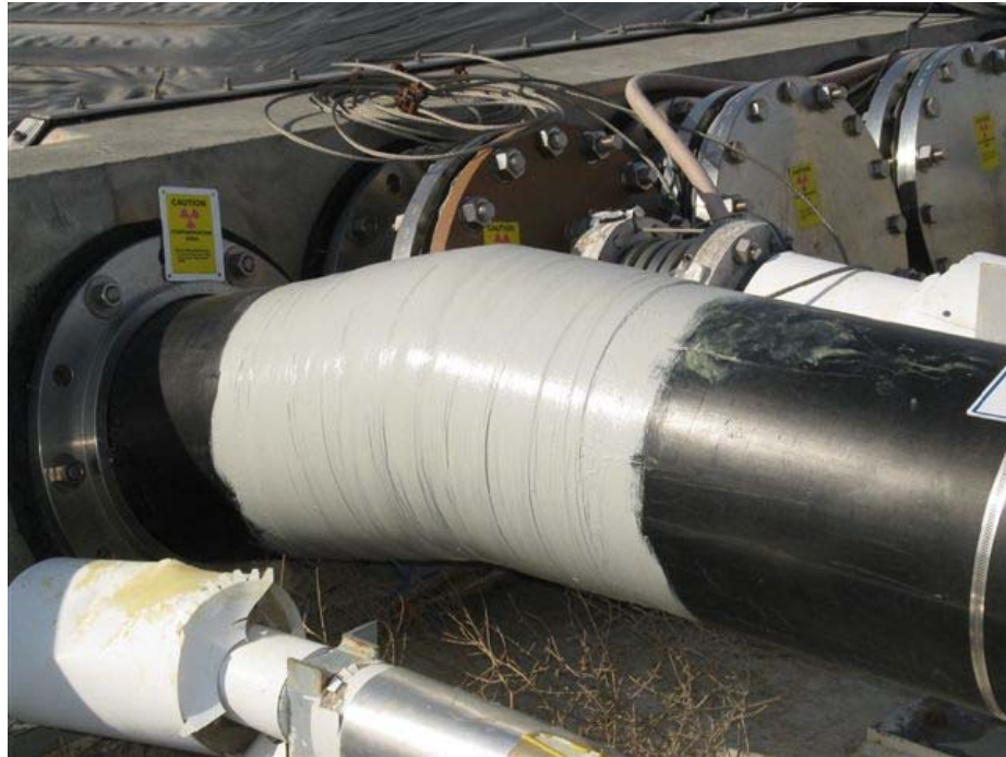
Fig. 4 – Final repair after paint coating
