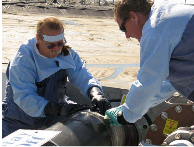
Fig. 2 – Application of epoxy impregnated base matrix to HDPE elbow
