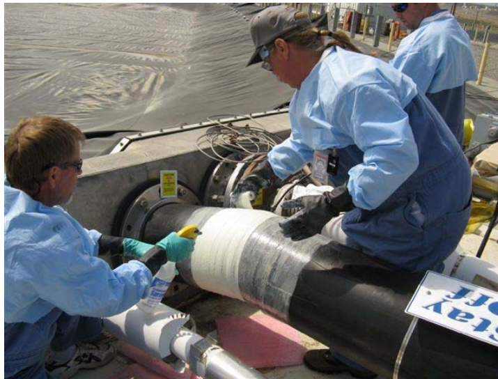
Fig 3 – Application of final layer as water activated fabric is wetted
