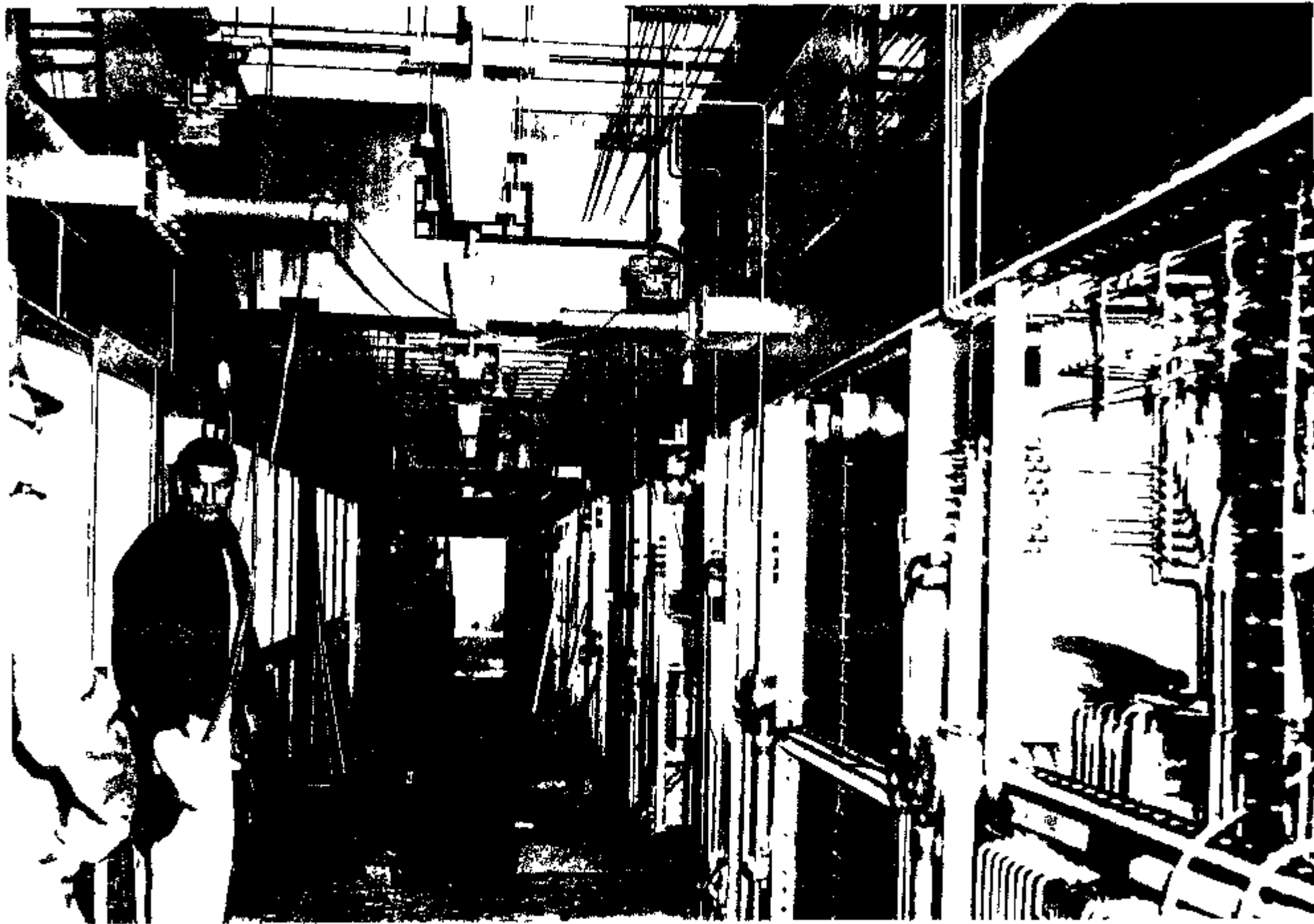
Figure 4 - Access Corridor for Equipment Maintenance and Replacement of HEPA Filters
