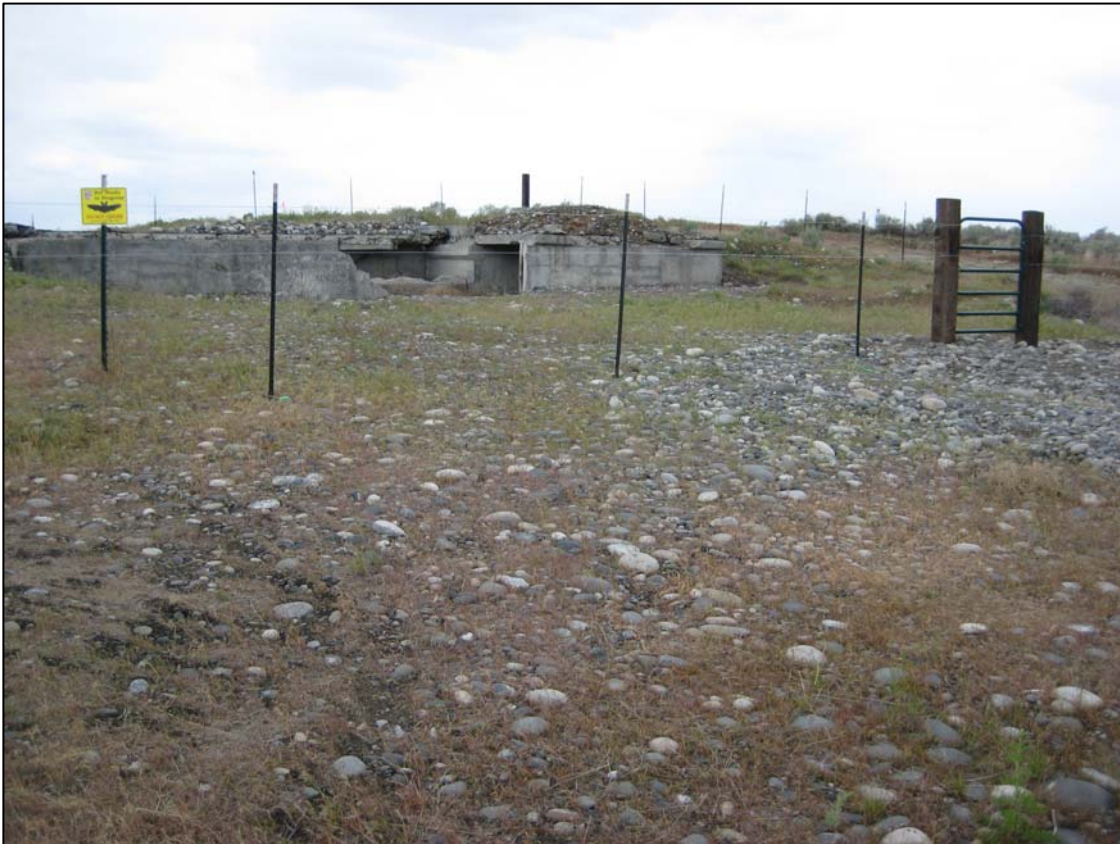
Figure 27. Fencing and Signage at the 183-F Flume Entrance.
