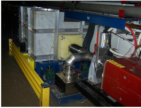
Figure 1: 20-Ton Secondary collimator
