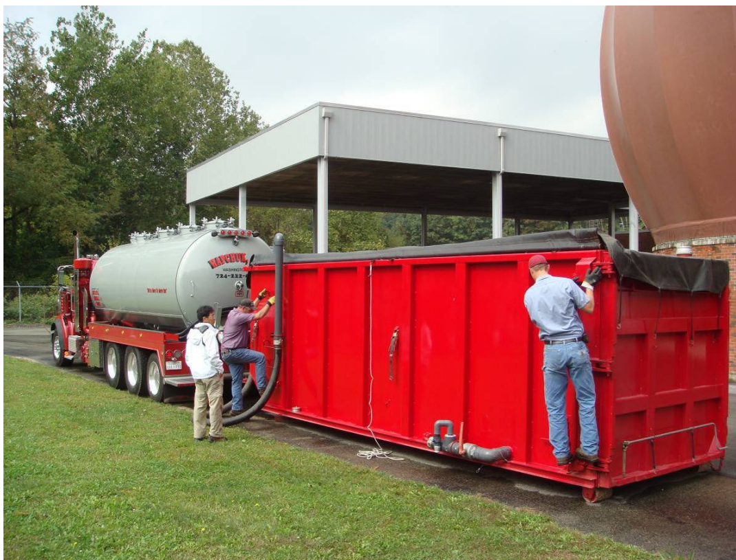
Figure E.15. The roll-off steel tank was placed on an asphalt surface next to the cooling towers at FTMSA. About 7000 gallons of treated AMD was stored and allowed to settle for 2 days before being used in the pilot-scale tests.
