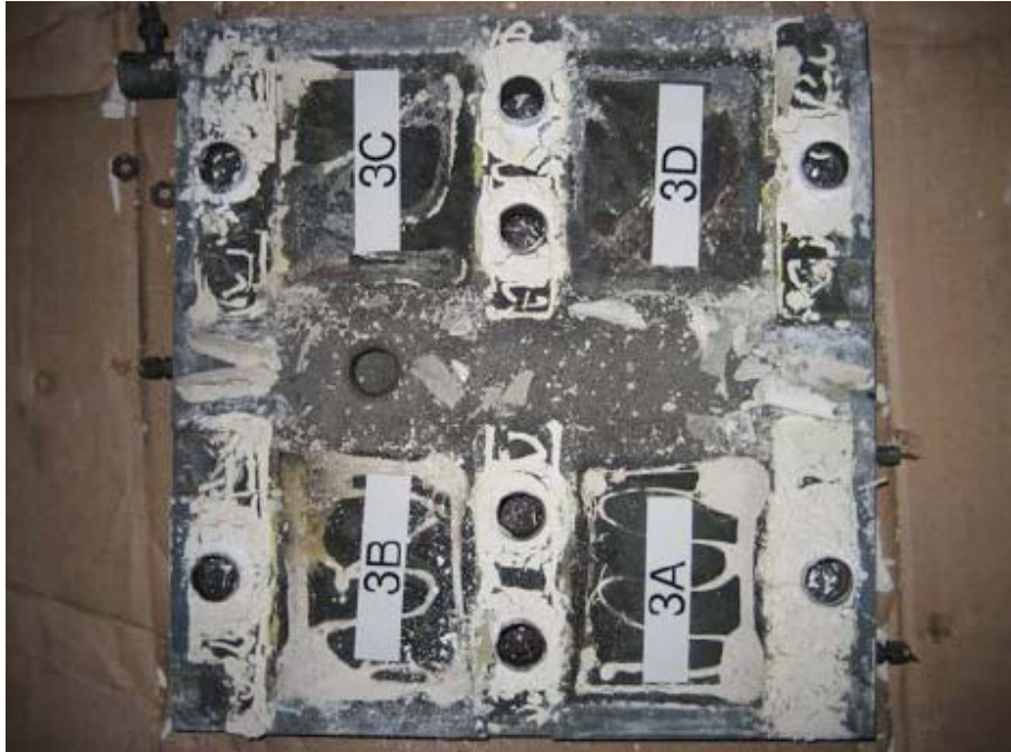
Figure 21. Module 3 base plate after stacks were removed.
