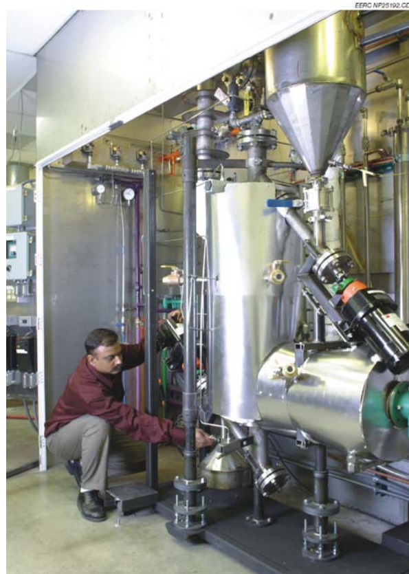
Figure 5. Photo of gasification system.
