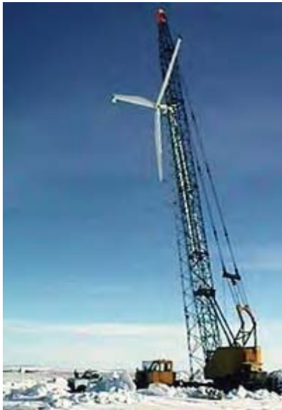
Erection of wind turbine at Kotzebue Electric Association.
