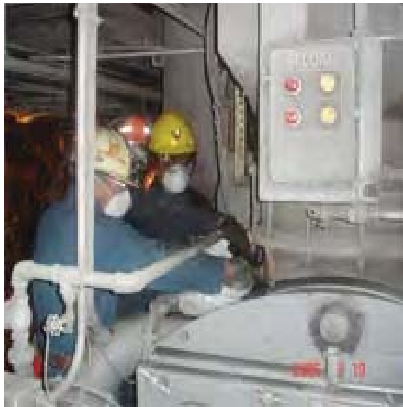
Figure 2.2. Raw (feed) coal sampling.
