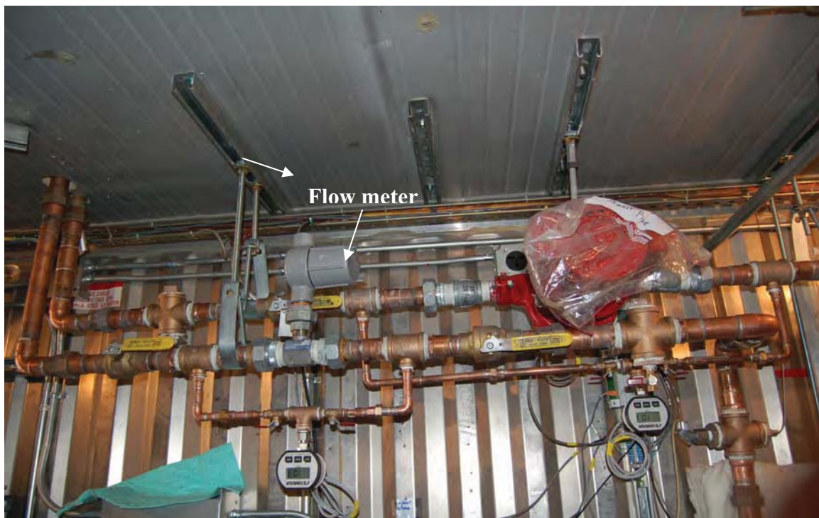
Figure 2.17. Flow meter line.
