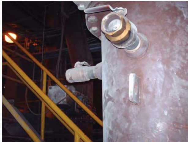
Figure 2.4. The perpendicular sampling ports.
