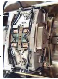
Photo: EMI pre-test module *1 ; finished
