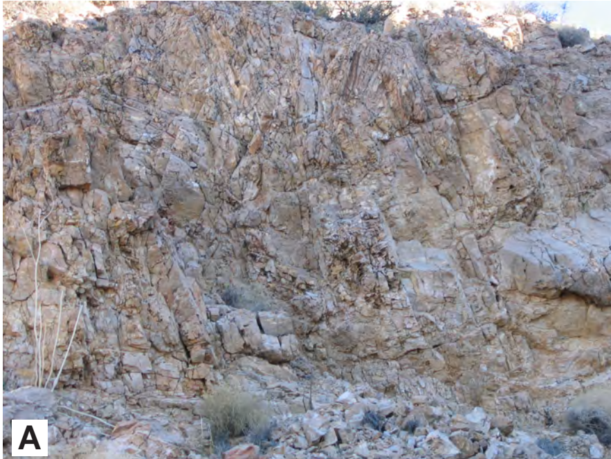
Intense fracturing of carbonate aquifer within damage zone on north side of fault at Station PR-65. Exposure is approximately 3.0 m (10 ft) high.
