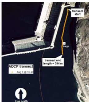
Figure D.13. Water Velocity Magnitude (top), Direction (lower) Collected on August 7, 2002, at 16:40 in the Forebay of the Third Powerplant at Grand Coulee Dam. In the plots, upstream is to the right, downstream to the left. The transect was along the centerline of the forebay (left). The directions in the lower graph are in an earth-referenced coordinate system (middle). Locations of turbine units 19 through 24 are indicated by vertical lines.
