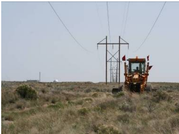
Figure 7. Road maintenance and archaeological resource avoidance during upgrades to the T-25 powerline access road.
