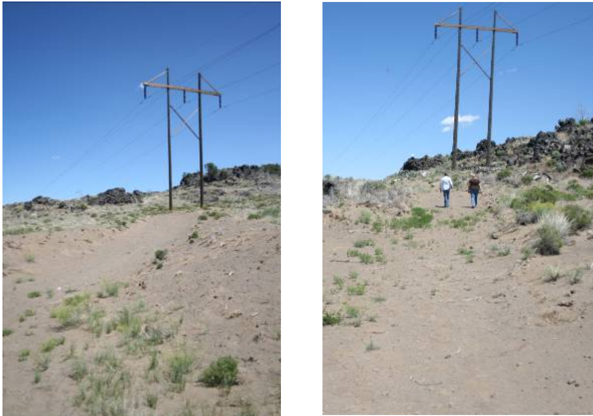
Figure 2. Type II impacts documented at 10-JF-135 (left) and 10-JF-88 (Hellofasite, right) from powerline maintenance. Note gravel fill beneath poles on the right.
