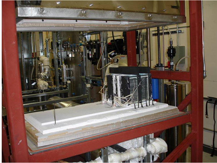
Figure 13. Hot zone enclosure with one module installed.
