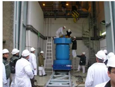
Figure 10. Specially designed cask-transfer device on rails in the High-Level Waste Storage Facility entrance hall.
