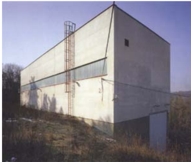
Figure 9. The High Level Waste Storage Facility.
