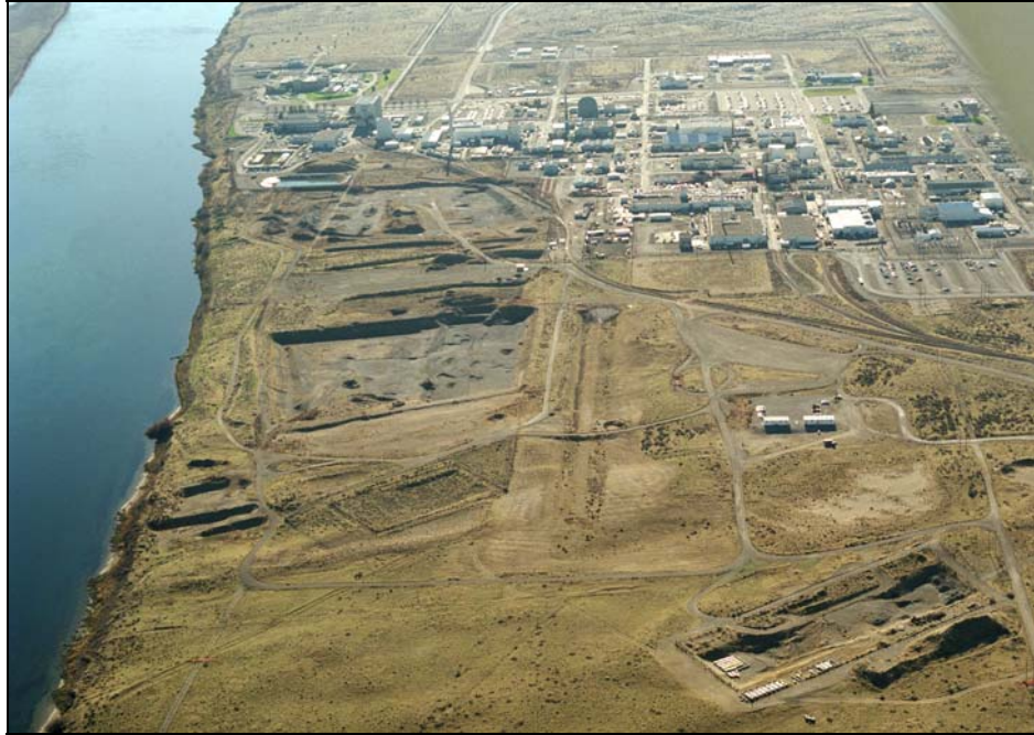
Figure 6.9. Aerial Photograph of 300-FF-5 Looking South with the Columbia River on the Left. The North and South Process Ponds (center-left) are partially excavated.
