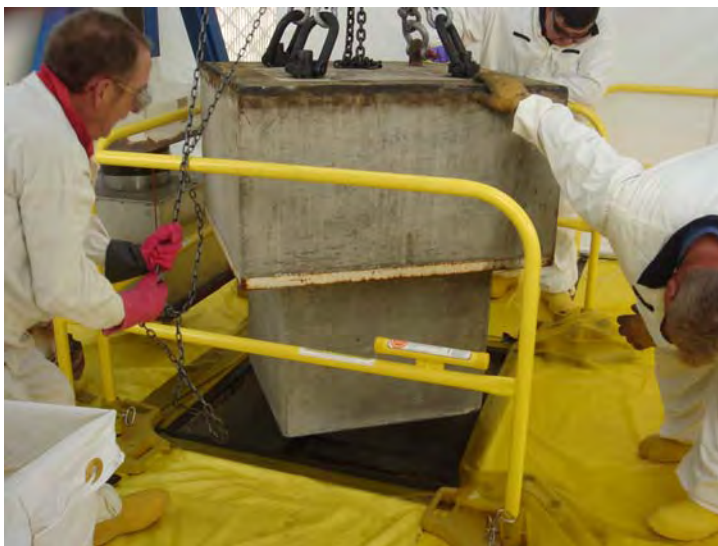
Figure 4.1. Vault Access Cover Block Removal
