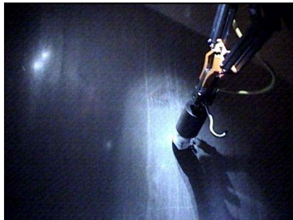
Illustration 50: Sampling - South Wall of A-Vault
