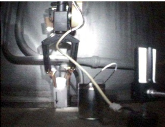
Illustration 56: A-Vault Sump Sampling
