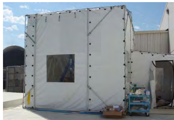
Figure 3.9. Containment Installed over HLV
