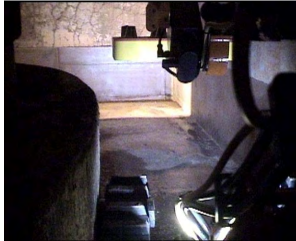
Illustration 26: Visual Inspection of B-Vault Southeast Corner
