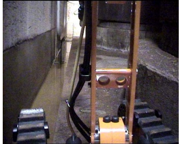
Illustration 14: Gutter and Sump as Seen by ROV
