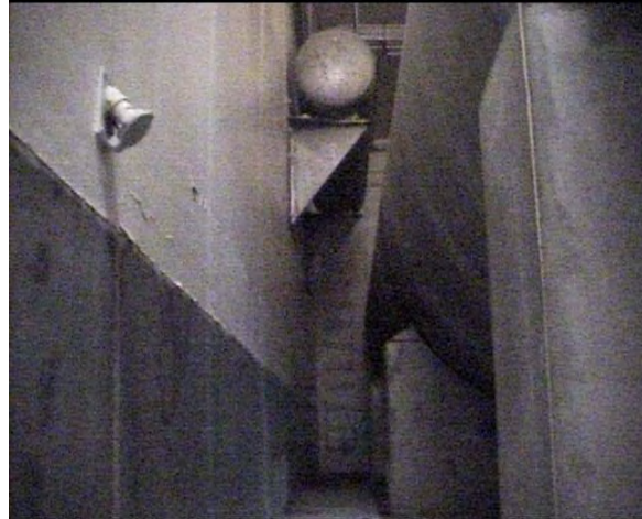
Illustration 42: ROV View of Tanks WT-1 and W-4
