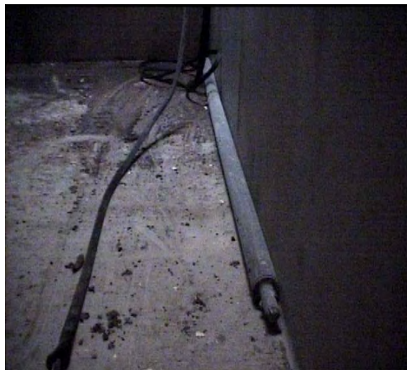
Illustration 69: Scaffold Tube on Floor
