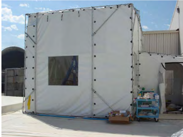
Figure C.13. Containment Installed over High Level Vault
