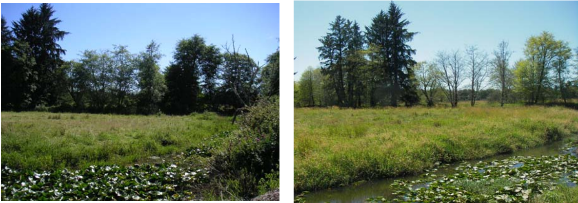
Figure 4.6. Before and After Photo Points at a Culvert Installation on Kandoll Farm
