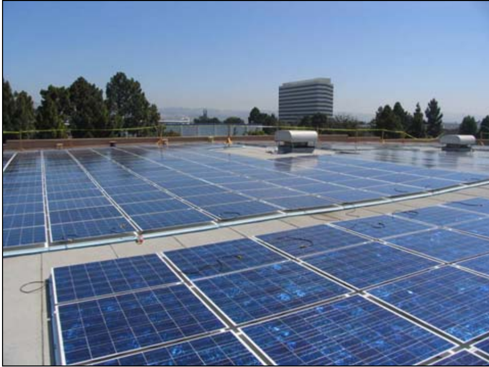
Figure 42: Demonstration array with reduced coating thickness during installation.
