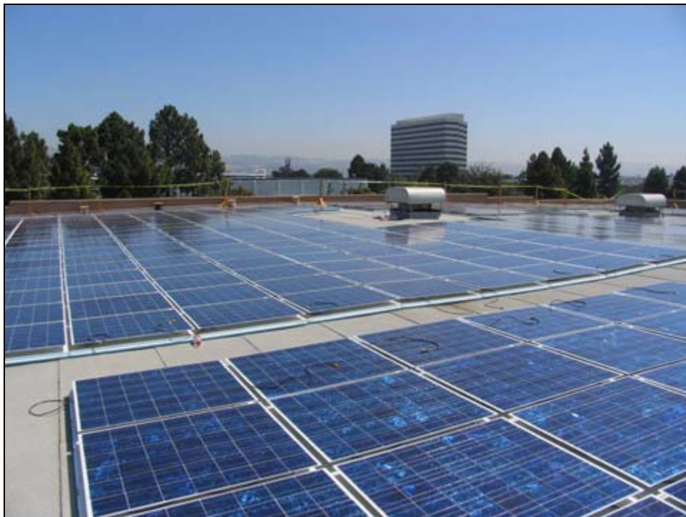
Figure18: New tiles installed prior to wiring.
