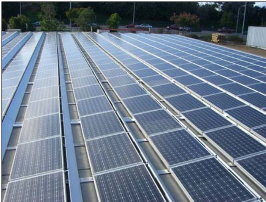
Figure 11: Completed Phase I RFT10 installation – 654 kWp system.
