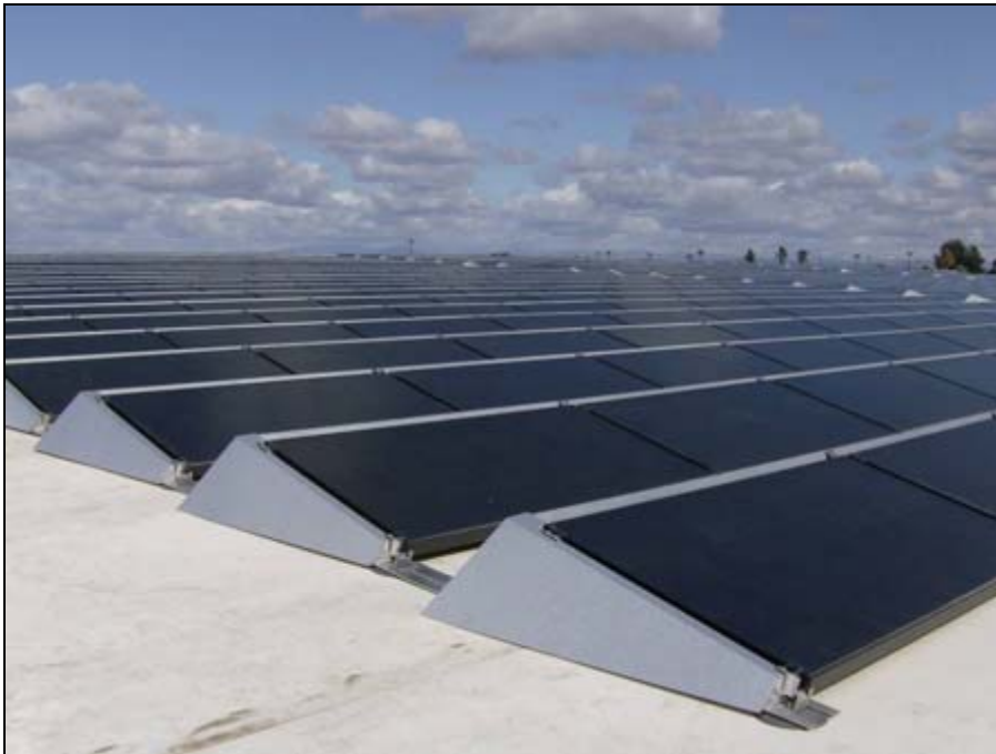
Figure 46: 1-MWp array completed.
