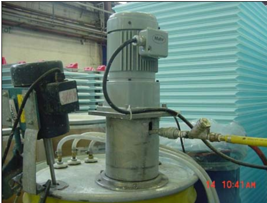
Figure 33: New pumping station for mixed liquids.
