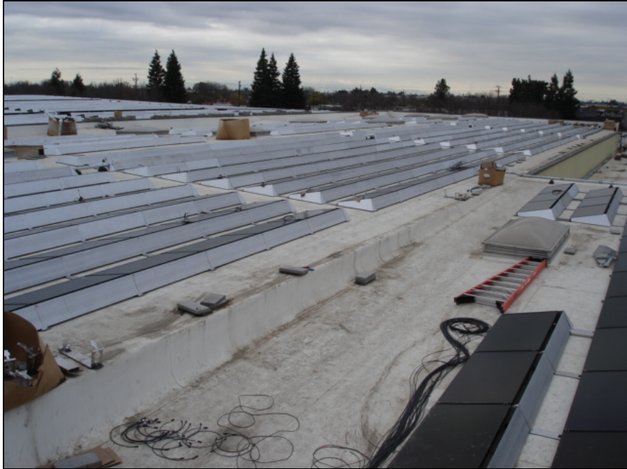
Figure 45: Commercial demonstration site under construction.
