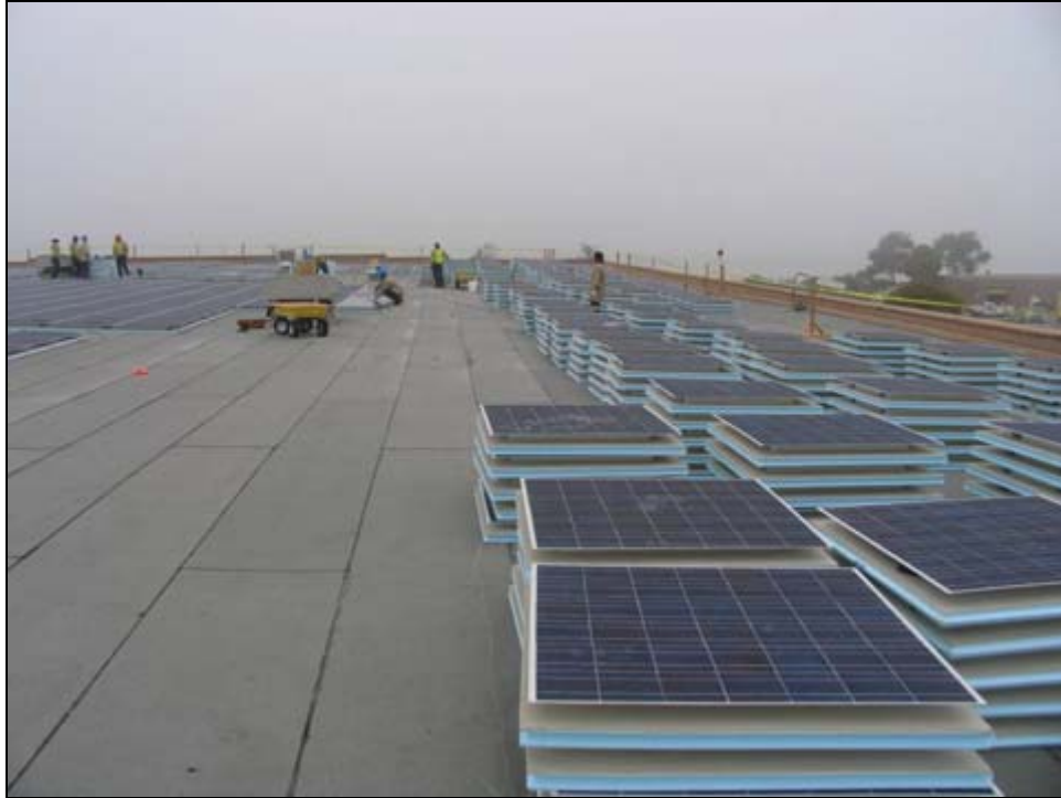
Figure 17: New tiles being installed.
