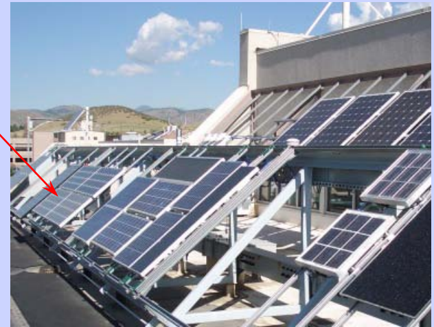
PERT: viewed looking west
