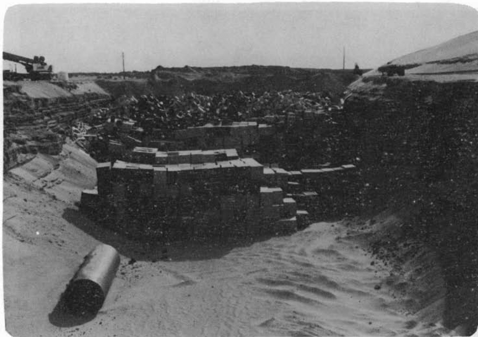
FIGURE 24. Use of Container Stacking for Radiation Shielding
