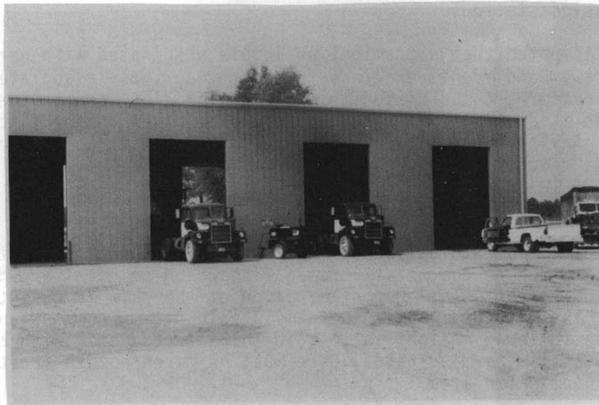
FIGURE 21. Cask Preparation and Maintenance Facility
