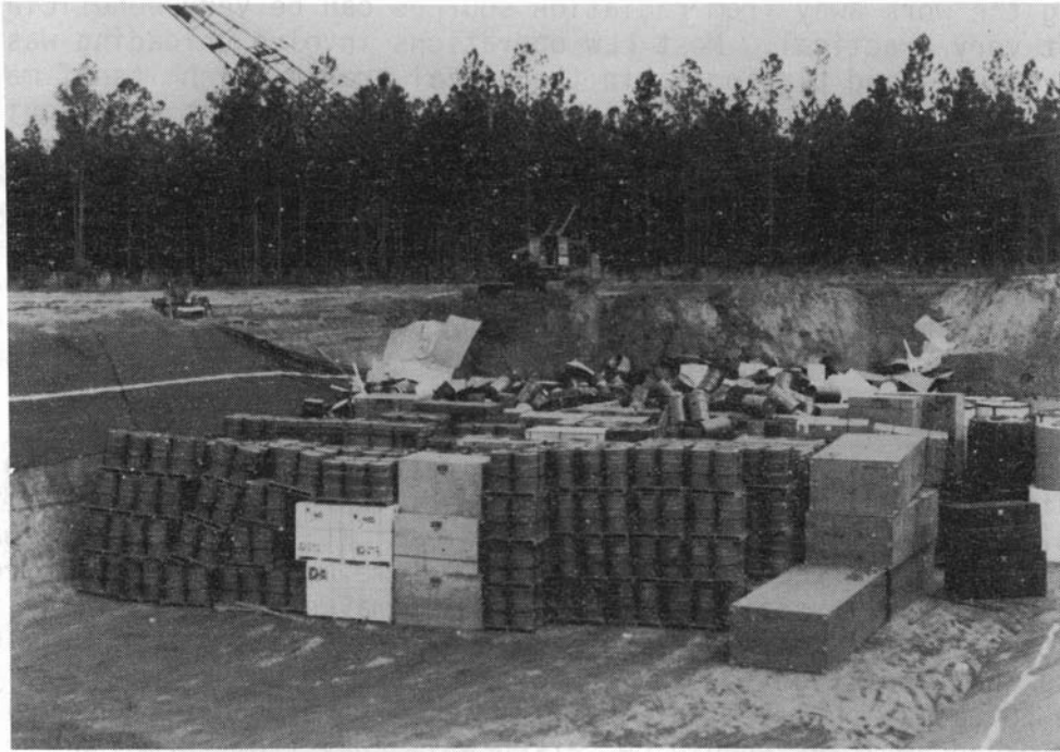
FIGURE 10. Shielding of Emplaced LLW Containers
