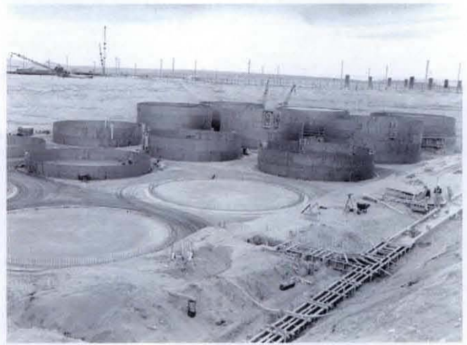
FIG. 2. 241-SX tank farm under construction.
