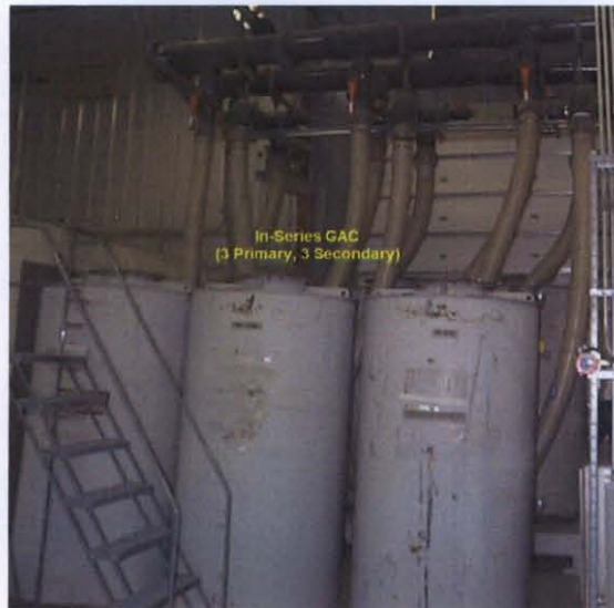
Figure 1-3. 200-ZP-1 Granular Activated Carbon Canisters (Total of Six Canisters).
