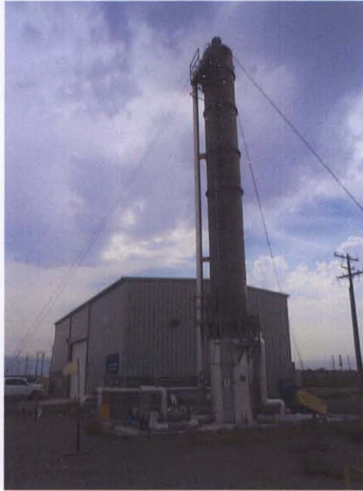
Figure 1-2. External View of 200-ZP-1 Facility.
