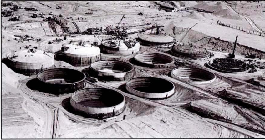
A Hanford single shell tank farm
