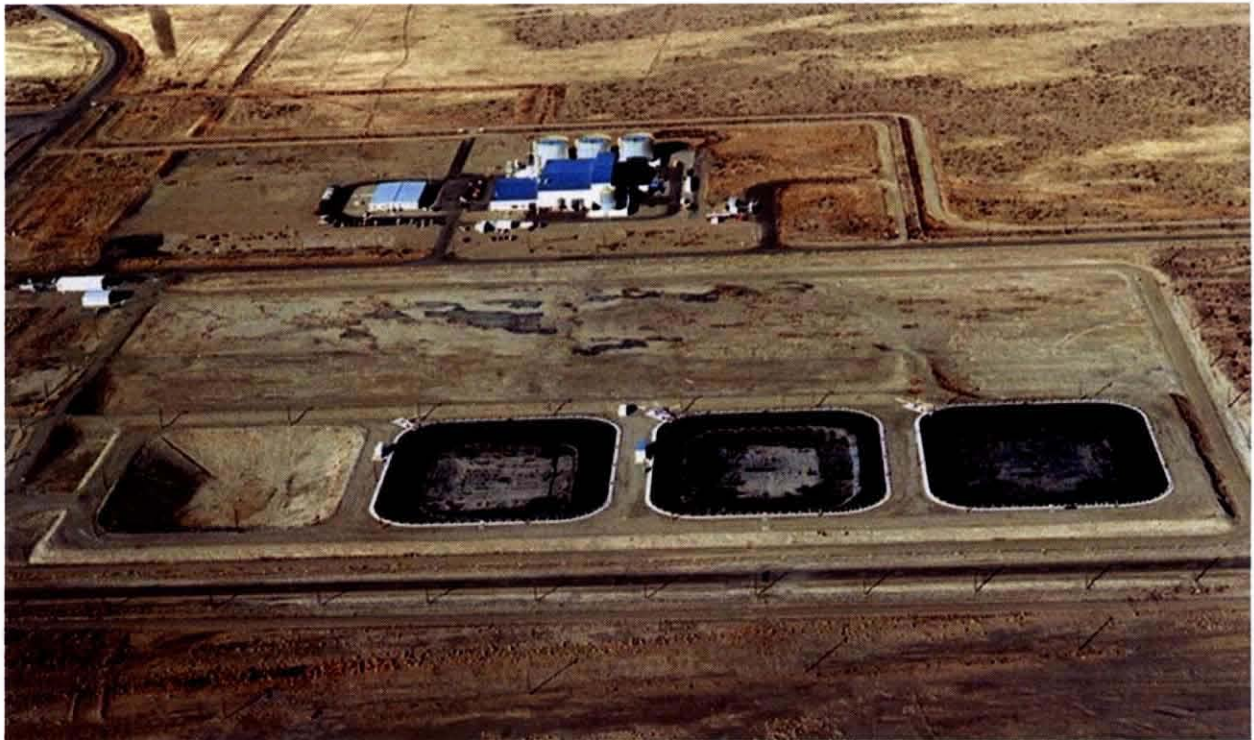
Hanford's Effluent Treatment Facility (ETF) – Used for the treatment of dilute waste streams.
