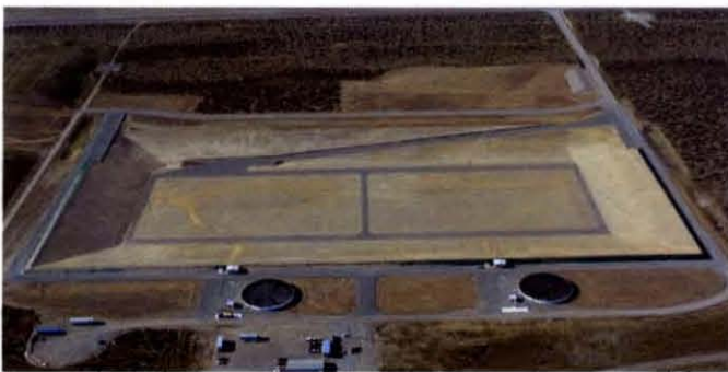
The Integrated Disposal Facility (IDF) – used for permanent storage of vitrified LAW and ETF solid waste.
