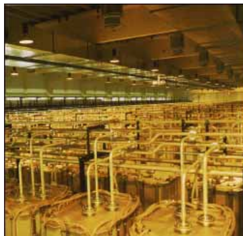
Fig. 19. Block-mounted centrifuges, Gronau.
