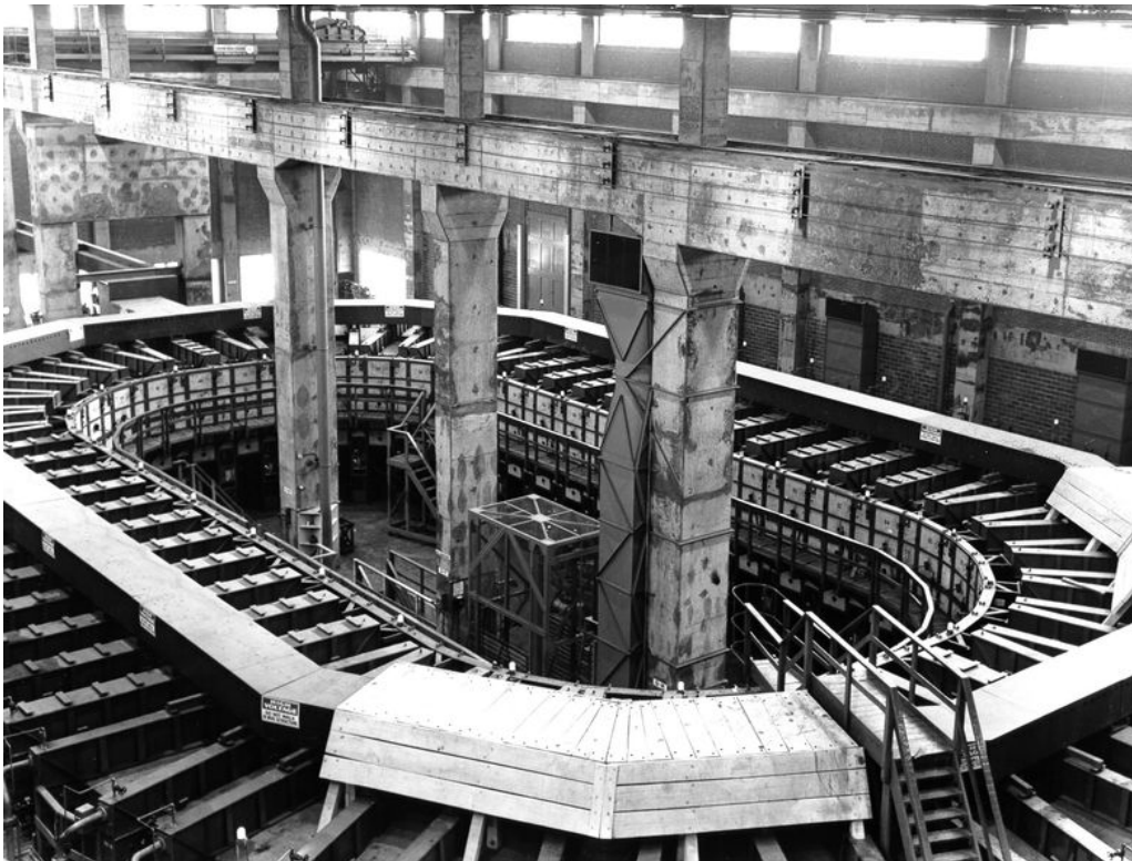
Fig. 1. Alpha Calutron track, Y-12 Plant, United States.
