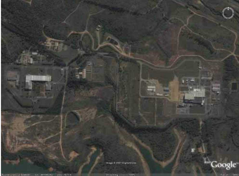
Fig. 25. Resende Nuclear Fuel Facility, Brazil.
