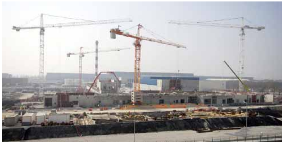
Fig. 17. Georges Besse II plant under construction, March 2007. 33
