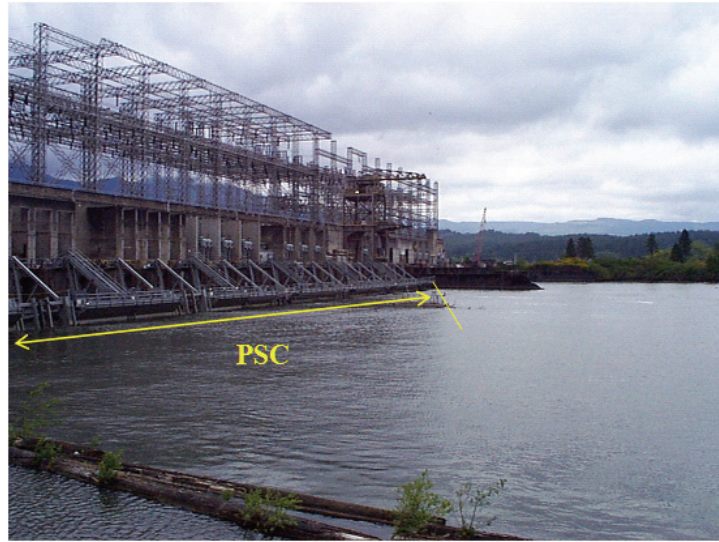
Figure 3.22. The Prototype Surface Collector at B1. (Photograph courtesy of M. Weiland)
