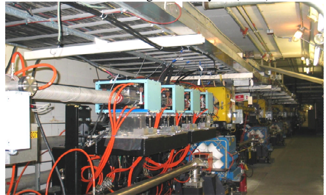
Figure 1. Detail of the newly installed 4-dipole chicane in the PEP-II LER in IR12 (upper beam line). The clearing solenoid can also be seen upstream of the first magnet (left side of the picture).
