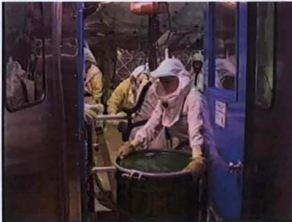
Removing Drum of Waste from Containment Tent
