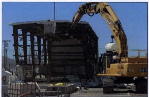
Excavator Pulling Down the 241-Z Structure
