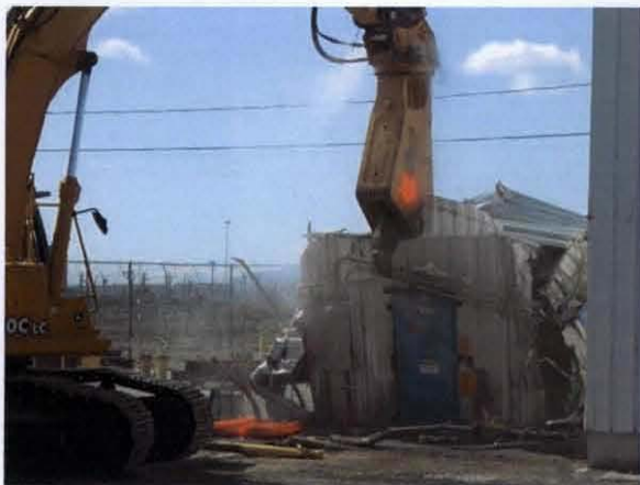
Demolition of 241-ZA Sample Building
