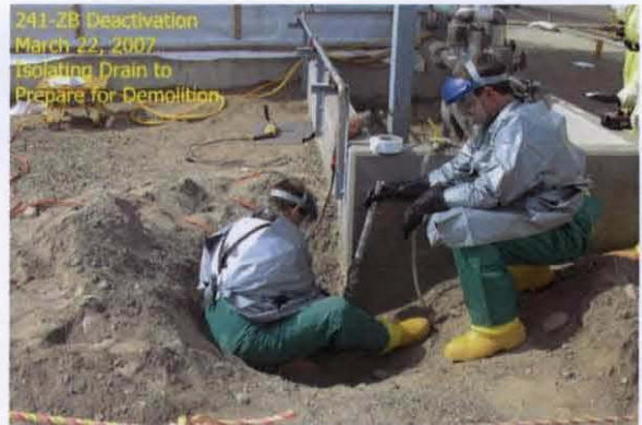
Cutting, Draining, and Capping a Buried Chemical Line to 241-ZB
