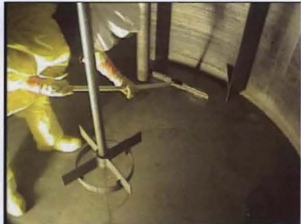
Cleaning Floor of a 241-Z Waste Tank
