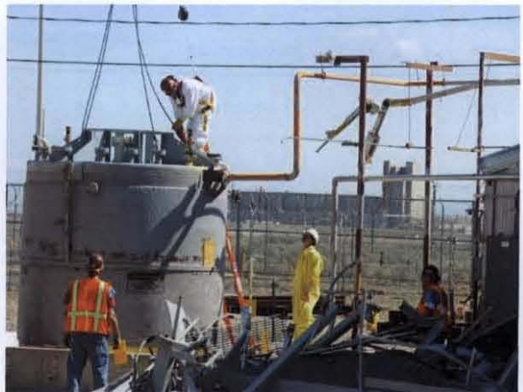
Rigging 241-ZB Caustic Tank for Removal from 241-Z Demolition Site
