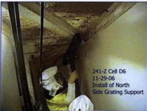
Installing Grating Reinforcement for Work Grating in Center Tank Vault
