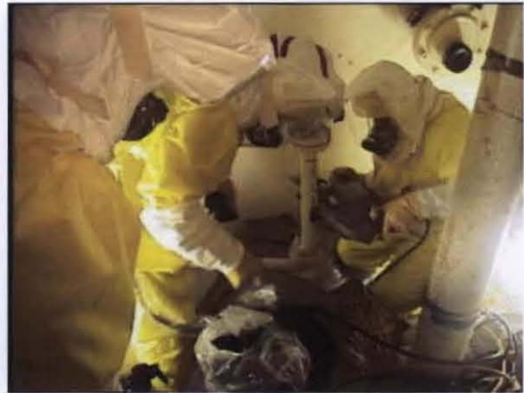
Size Reducing Process Pipe in 241-Z Tank Vault (Work Grating Level)
