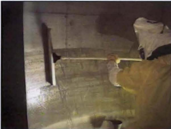
Cleaning Interior Wall of a 241-Z Waste Tank
