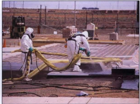
Installing Polyurea Environmental Barrier on 241-Z Slab
