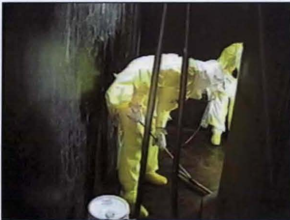
Cleaning a 241-Z Tank Vault Floor
