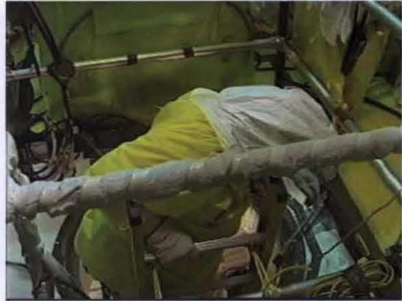
Worker Entering 241-Z Tank Vault Via 39" Opening
