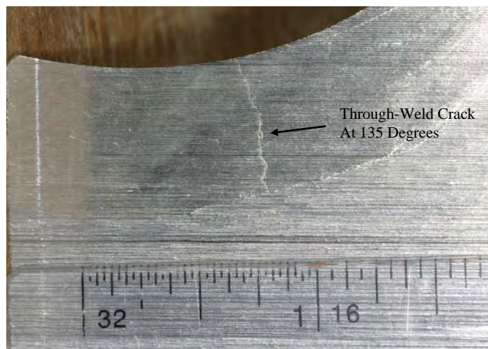
Figure 6.12. Confirmed Through-Weld Crack Found Above the Triple Point in Section 2 at 135 Degrees
