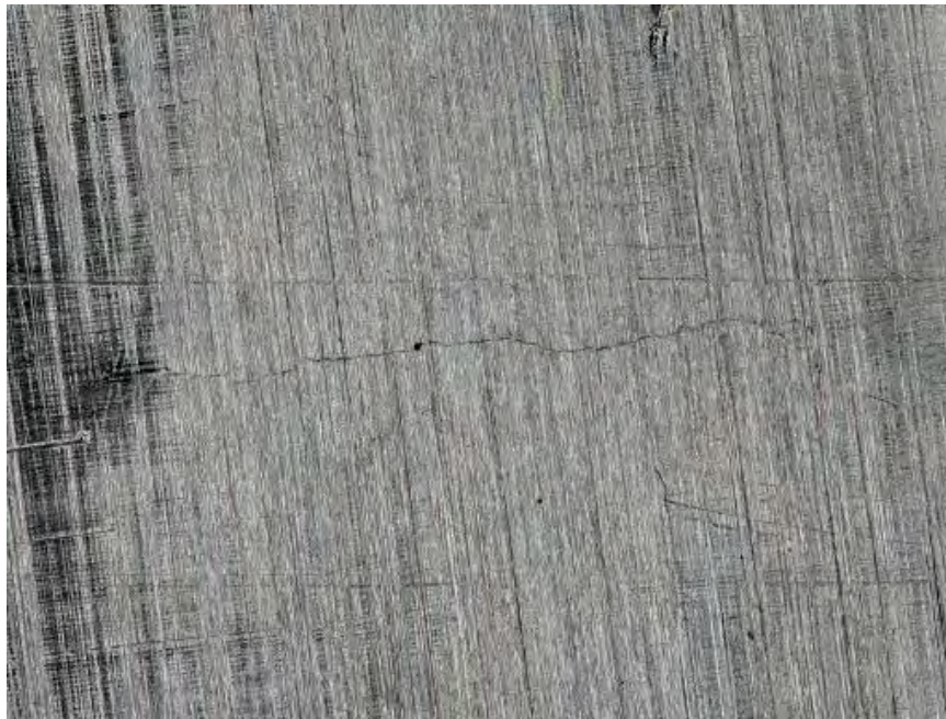
Figure 4.14. A Crack 28 \mu\text{m} (0.001 in.) Wide Cutting Perpendicularly Across Machining Marks
