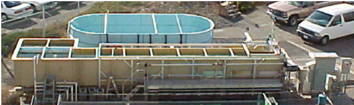
Figure 3.1. Test flume (shown in foreground).
