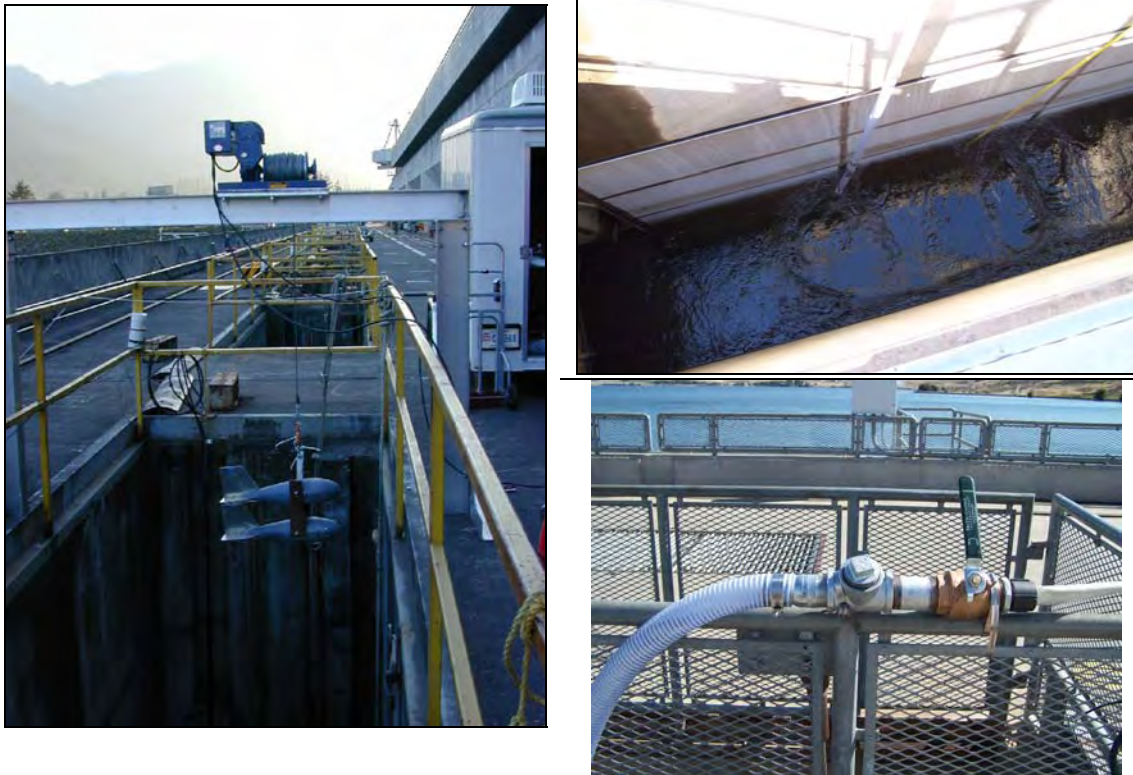
Figure 3.5. Sensor Fish induction system. Left photograph shows the winching system with sounding weights attached; right top photograph shows the induction hose routing down into the turbine gate slot; right bottom photograph is the ball valve, which controls the supply of water to the Sensor Fish induction system.
