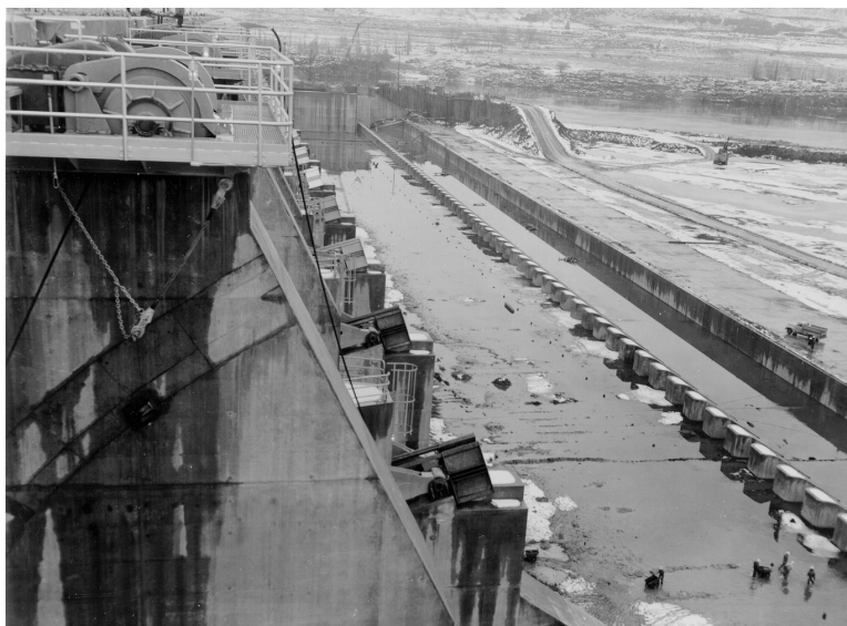
Figure 1.7. Photograph taken during the construction of The Dalles Dam. The photo shows the stilling basin, baffle blocks and endsill.
