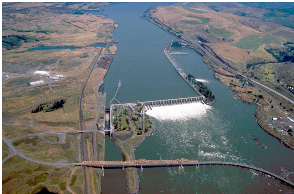
Figure 1.4. Aerial view of The Dalles Lock and Dam with all spillway bays operating.
